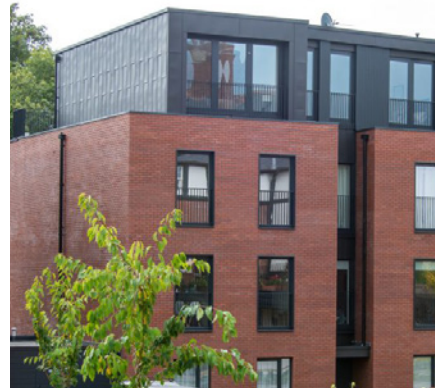
Zinc cladding to upper levels.
