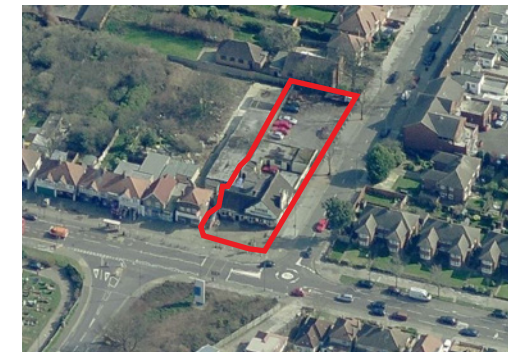
4. Site boundary west view
