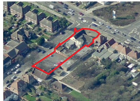
2. Site boundary east view
