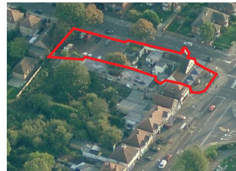
3. Site boundary north view
