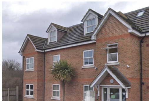
Neighbouring 3 storey residential building with dormers.
