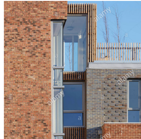
Combination of red brick and curtain walling.
