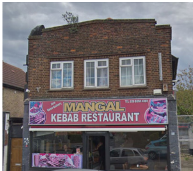
High parapet of neighbouring property on Hanworth Road.
