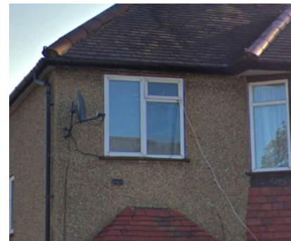
Window sizes in keeping with local residential buildings.
