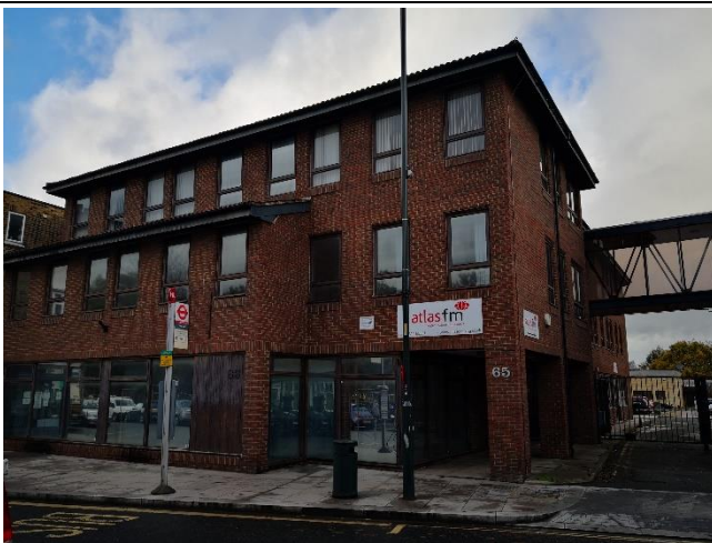
FIGURE 1: FRONT VIEW OF EXISTING BUILDING
