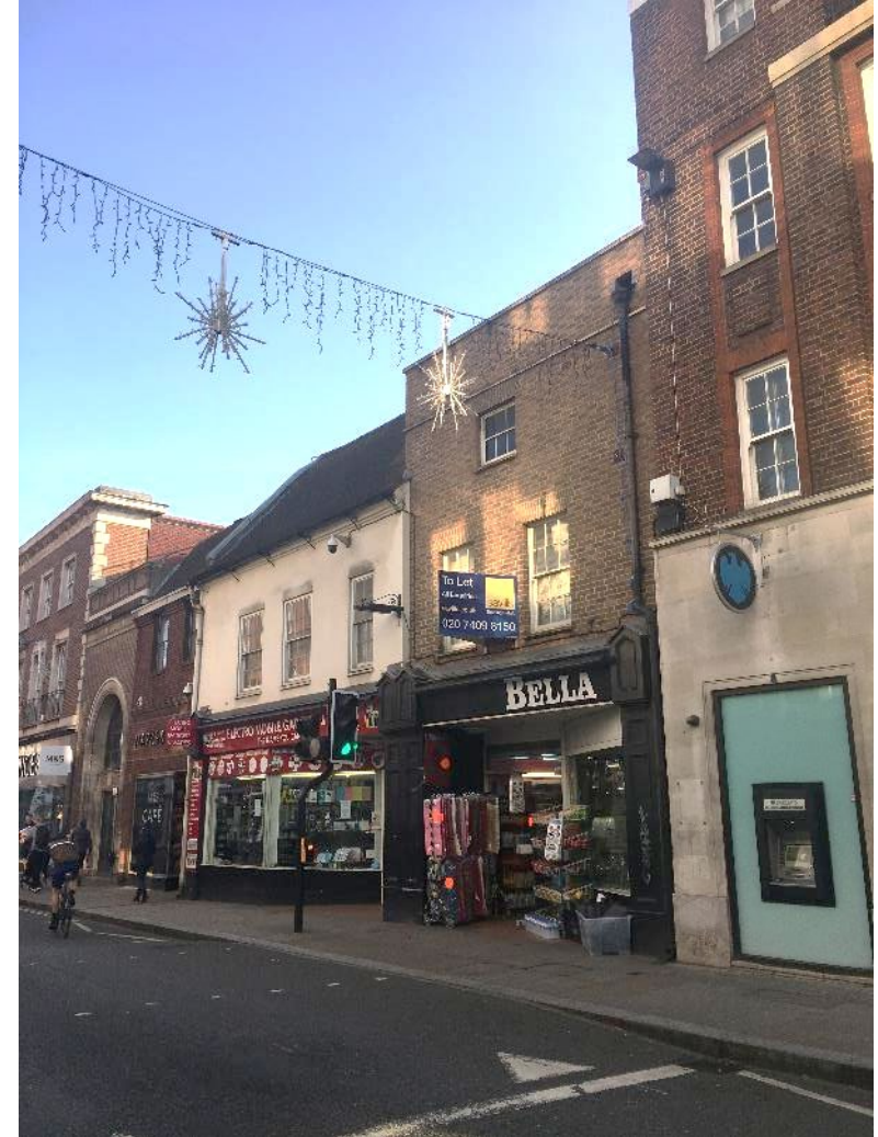
Plate 4: Front elevation from street-level.
