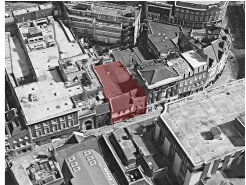
Plate 2: Aerial view of the front elevation and roof.
