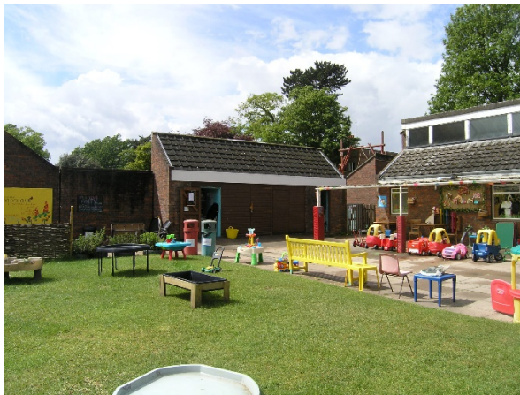
Looking northwest at the existing building (One O'Clock Club)
