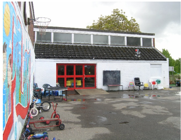
Looking south at the existing building (Adventure Play facility)
