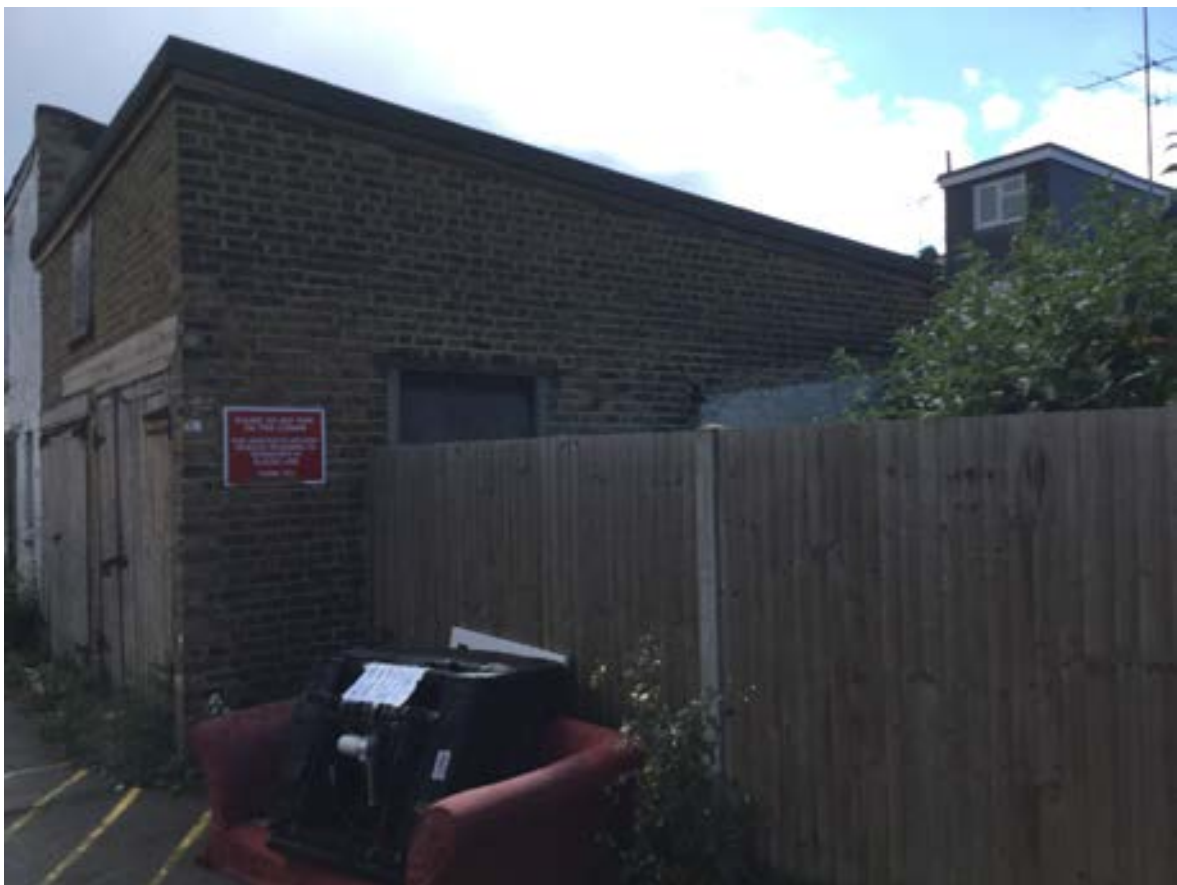
Plate 2: View looking east at the western part of the site
