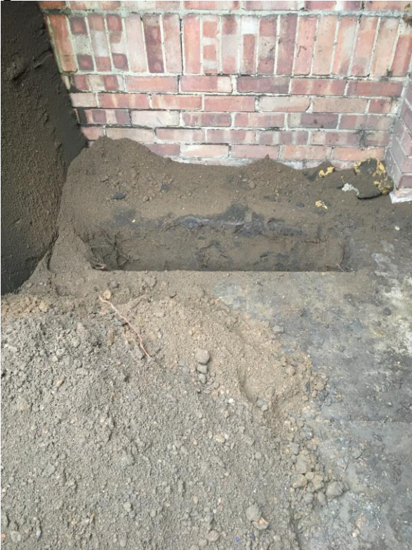
Fig 3. Trial trench 2 by front wall, shed to left of image
