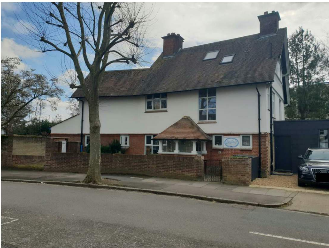
Similar porch roof proposed on 2a Cole Park Road as 4 Cole Park Road
