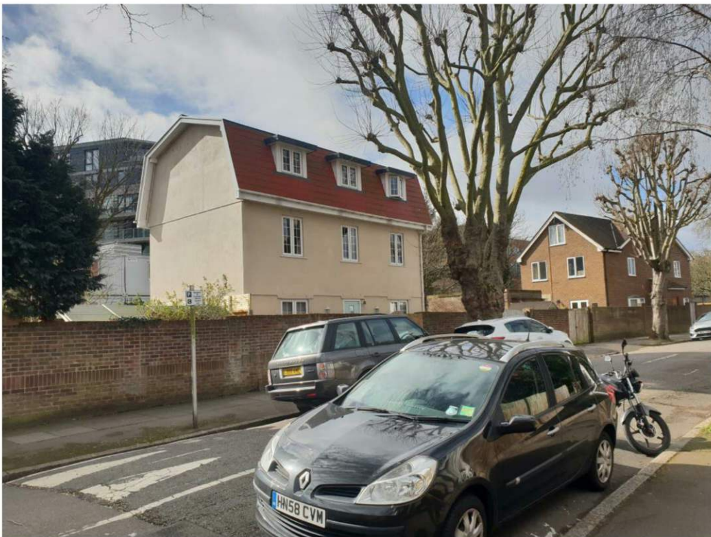
View of 3 storey gambrel roofed house at 2c Cole Park Road
