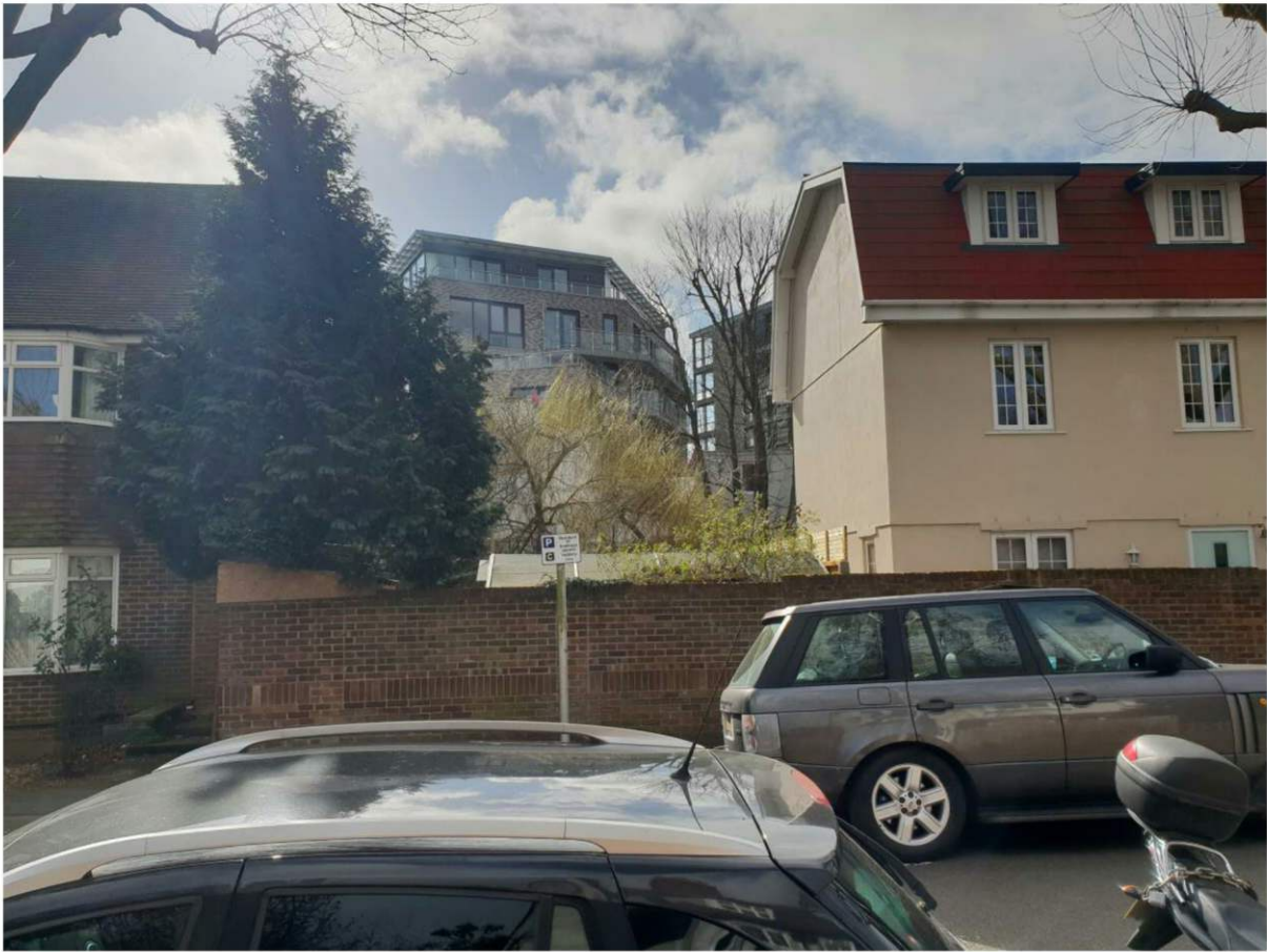
Modern flats are still visible in the retained gap between 2a and 2c Cole Park Road
