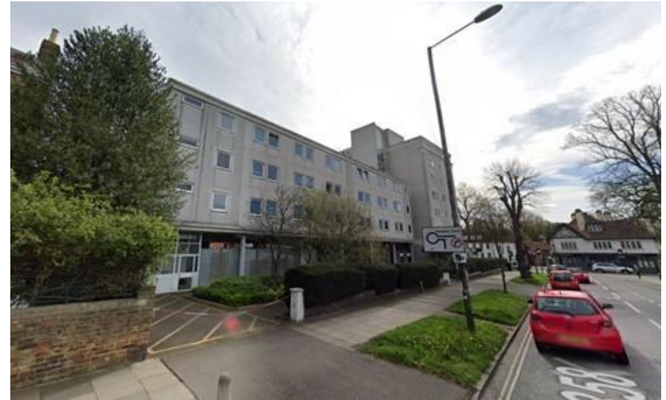
Elevation onto Grove Avenue
