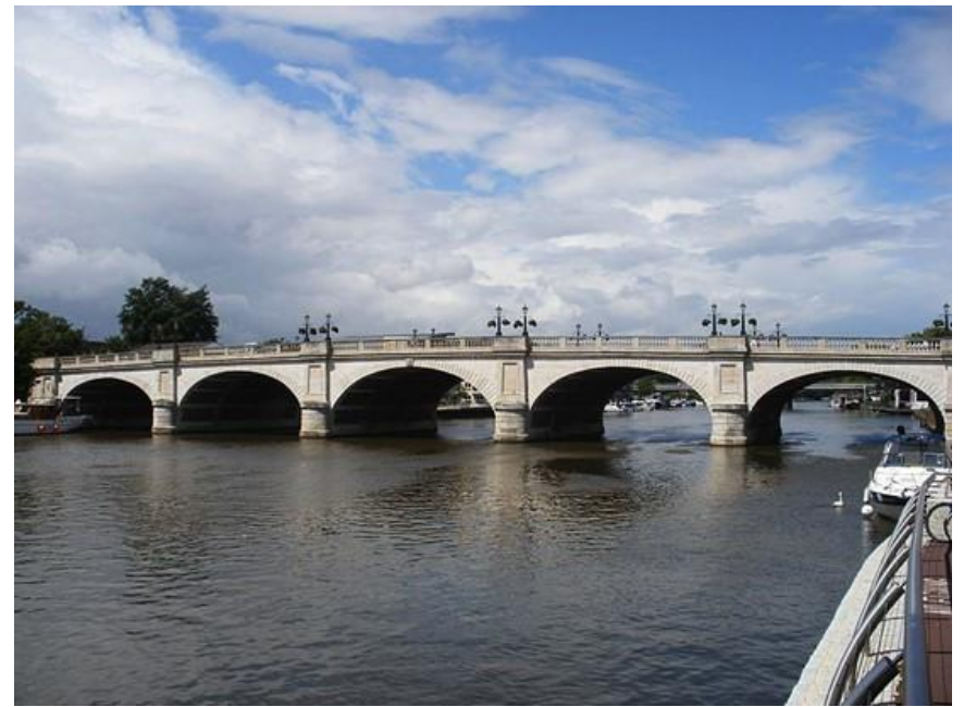
Grade II* Kingston Bridge
