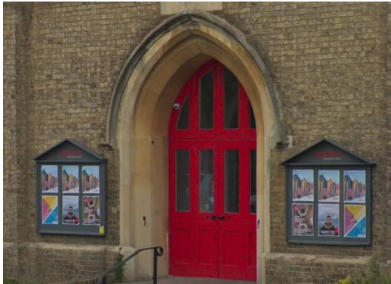
Stone arch and yellow stock brick church
