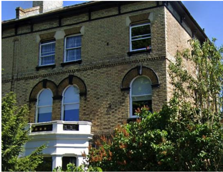
Yellow brick window surrounds and details.
