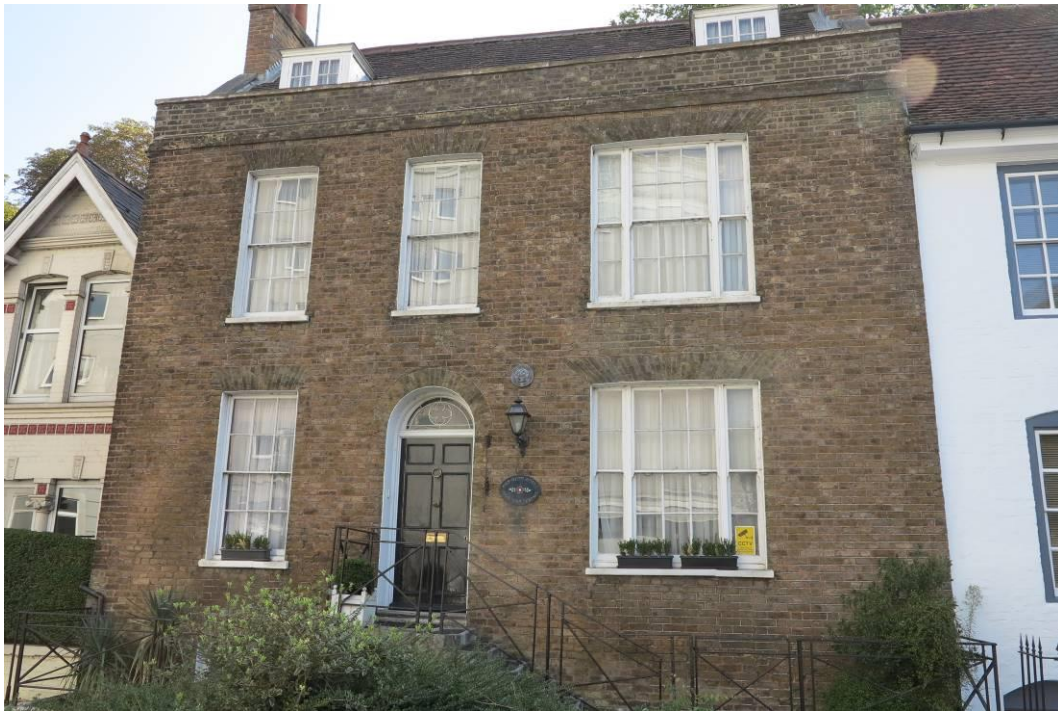
Plate 11. Home Park Terrace – the Gate House
