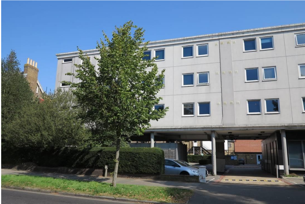
Plate 3. The northern range of Kingston Bridge House from the west
