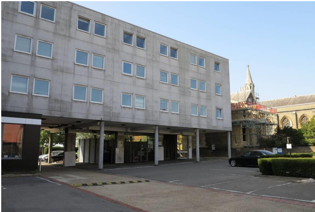
Plate 7. The rear of the northern range of Kingston Bridge House
