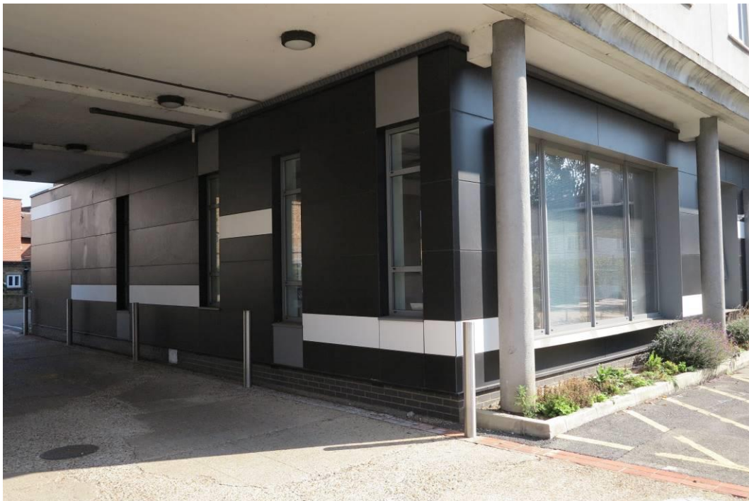
Plate 4. The undercroft has been partially infilled in the 1990s
