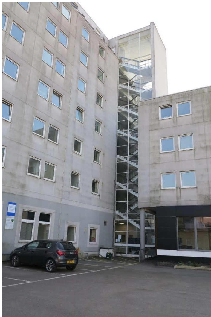
Plate 6. The stair core from the rear
