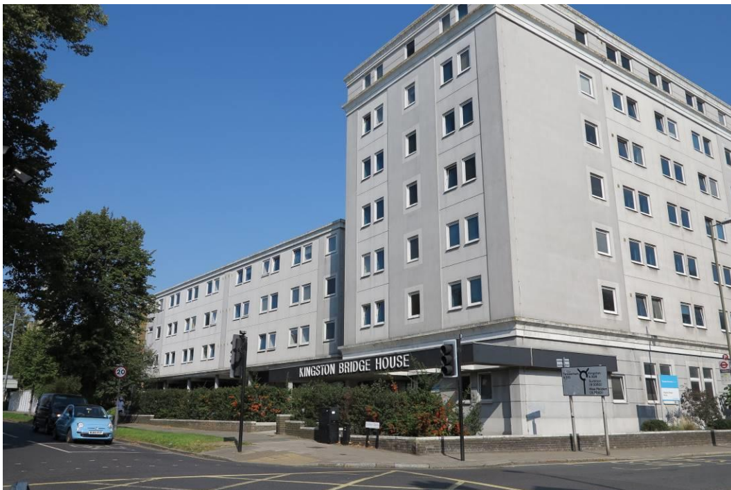
Plate 2. Kingston Bridge House from the south-west
