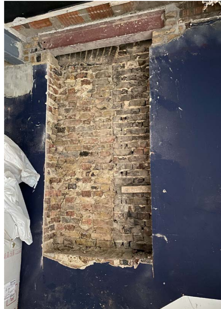
Figure 4.11 Blocked window on the south-west elevation of the original building..
