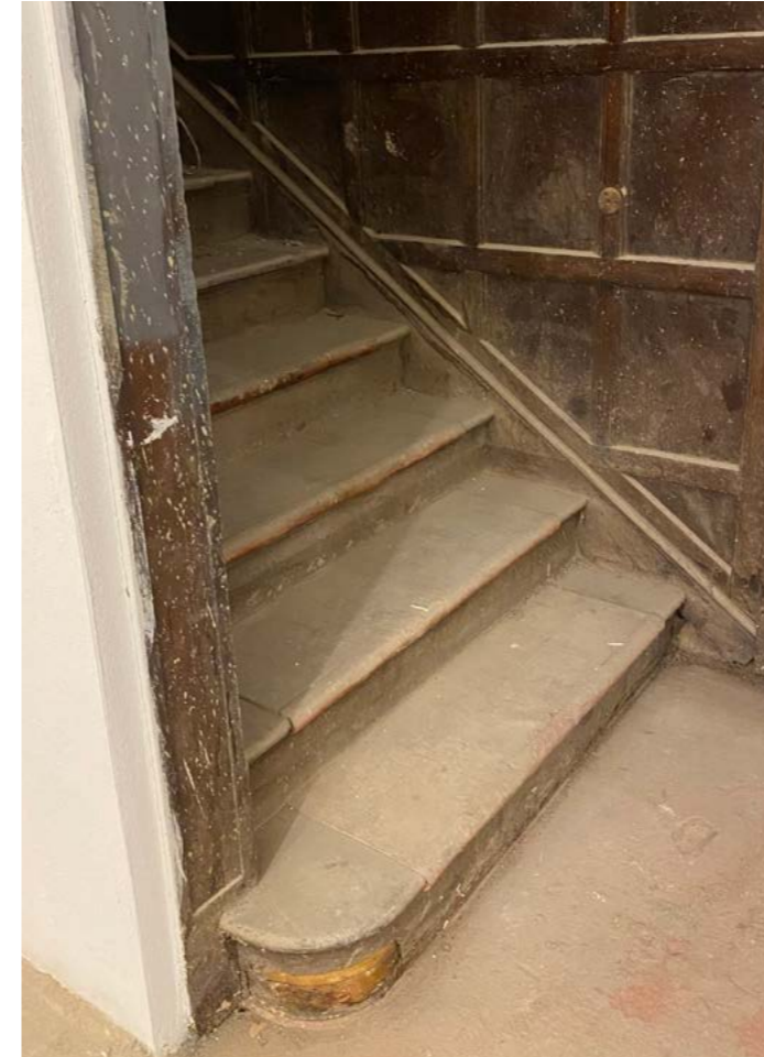
Figure 4.7 . Staircase with bull-nosed treads.
