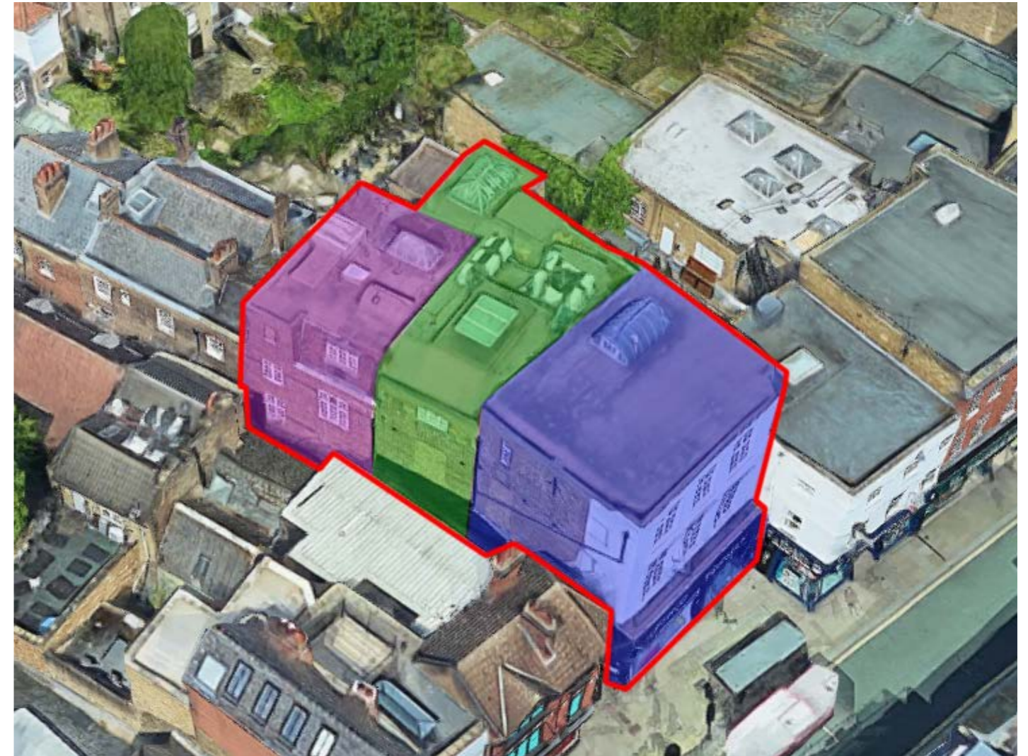
Figure 4.1 Aerial photograph of the Site. The Site boundary is marked in red. The early-nineteenth century (original) building facing George Street is coloured blue. The central building, constructed in the late-nineteenth century is coloured green. The north building, constructed in the late-nineteenth century is coloured purple.
