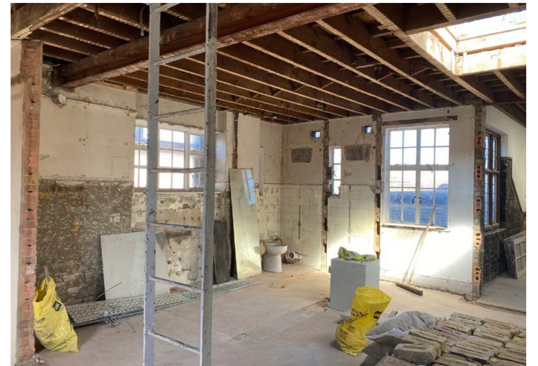
Figure 4.16 The second floor level of the north building, facing north-east.
