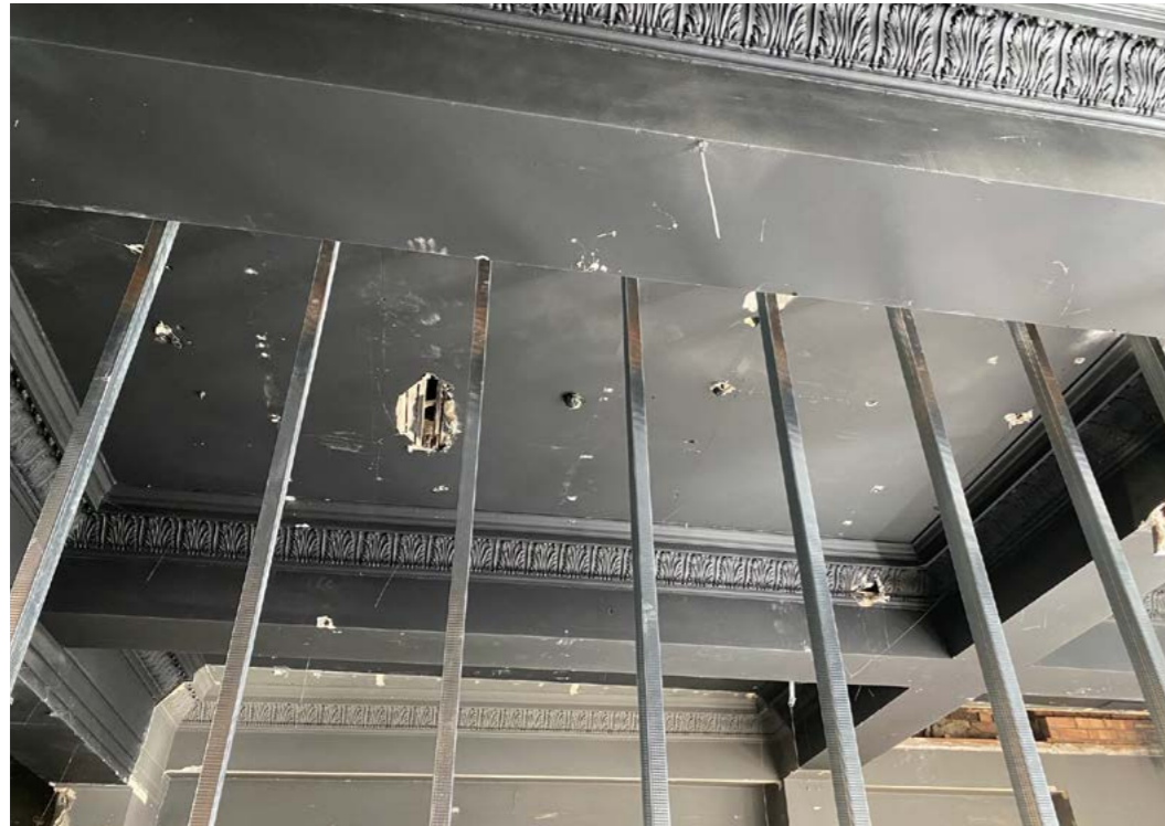
Figure 4.9 Modern ceiling treatment at first floor level.
