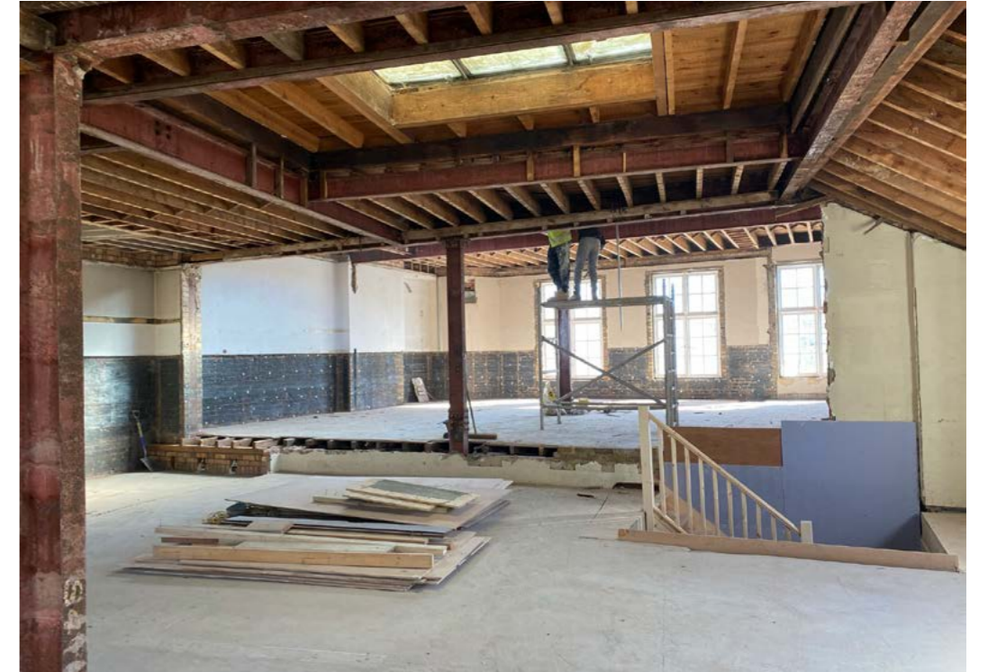
Figure 4.15 The second floor level of the central and original buildings.
