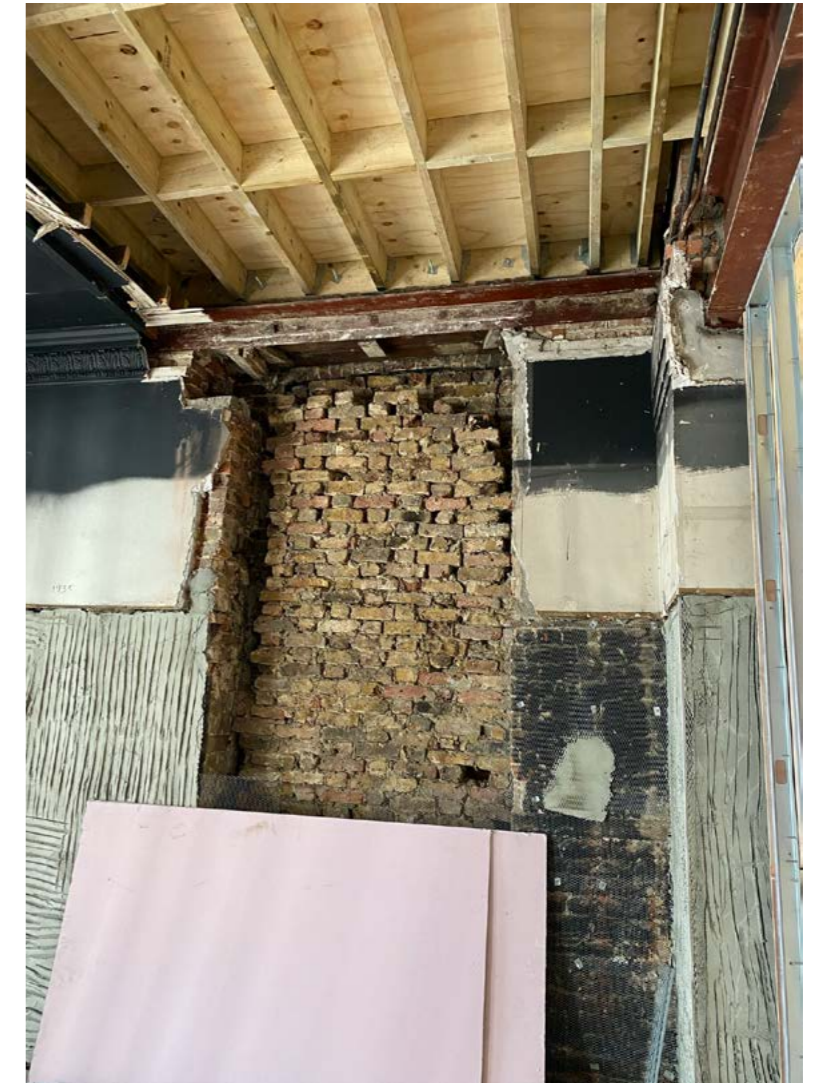
Figure 4.12 Blocked window on the south-west elevation of the central building..
