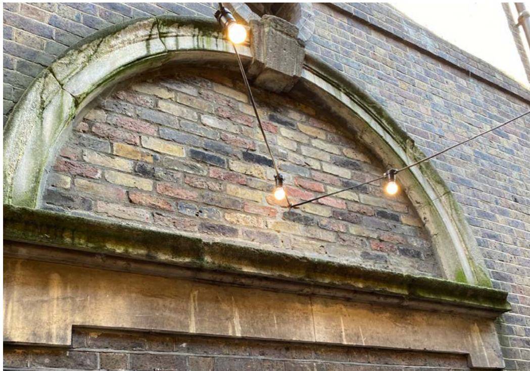
Figure 4.3 Stone arch at ground floor level on the south-west elevation.
