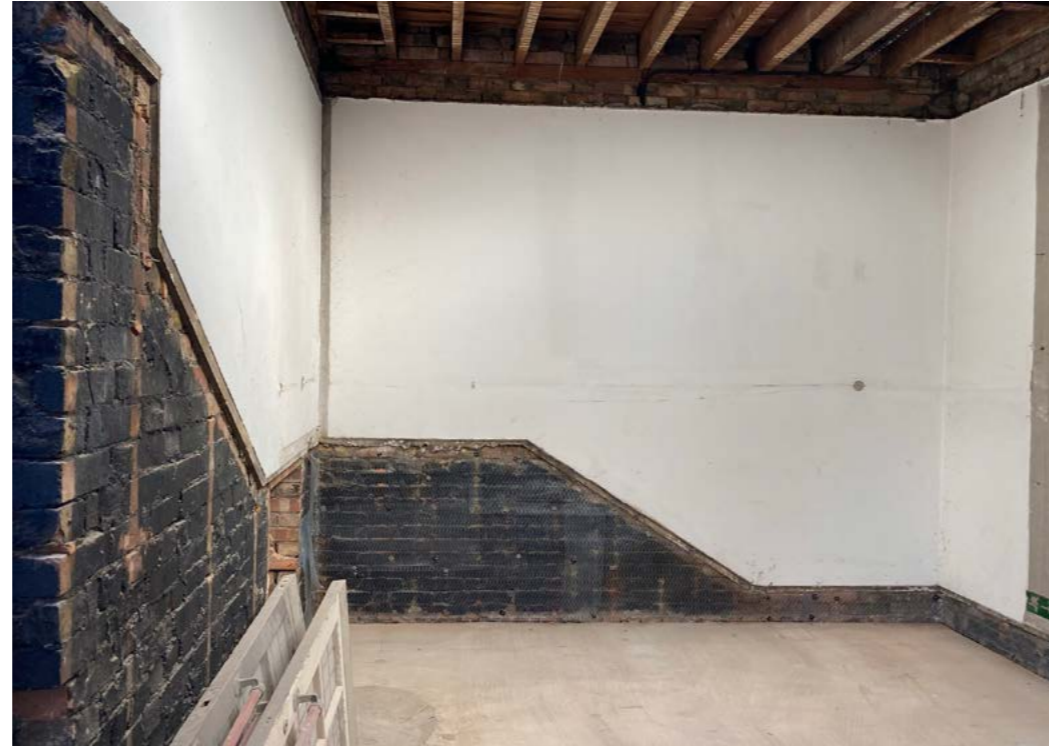
Figure 4.13 Evidence of a historic staircase at second floor level.
