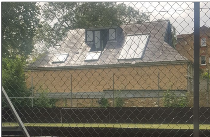
Figure 5 – Southern elevation of No. 64a Kings Road looking onto the Site
