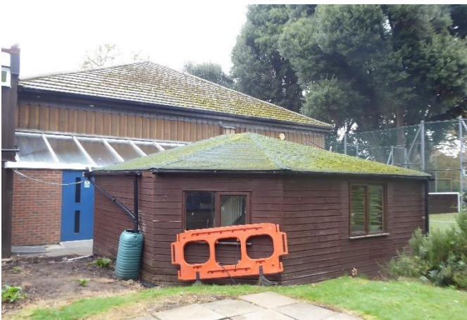
Figure 6.3: Photograph of the existing external store
