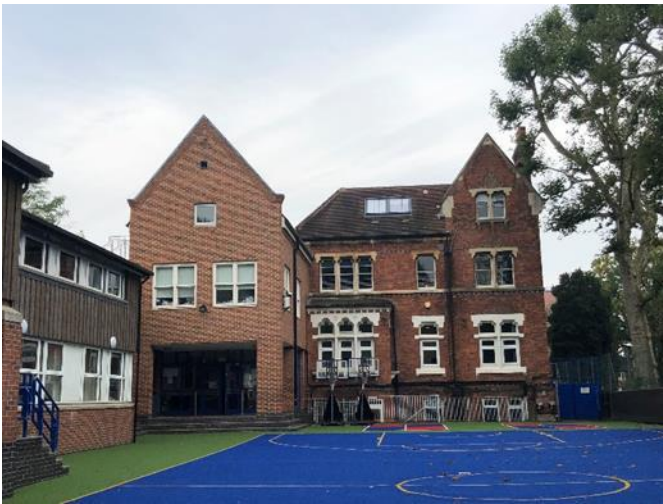
Plate 6: Rear elevation of No. 68 Kings Road, looking west
