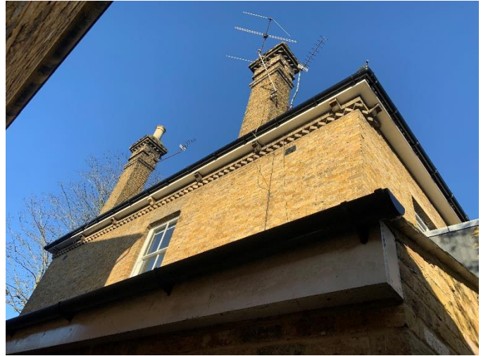
Photograph 7 Southern elevation of B1.2 and B1.8.
