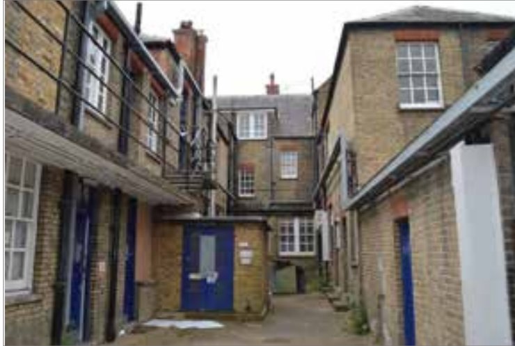
The rear of the building
