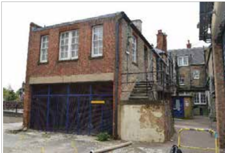
The rear of the building
