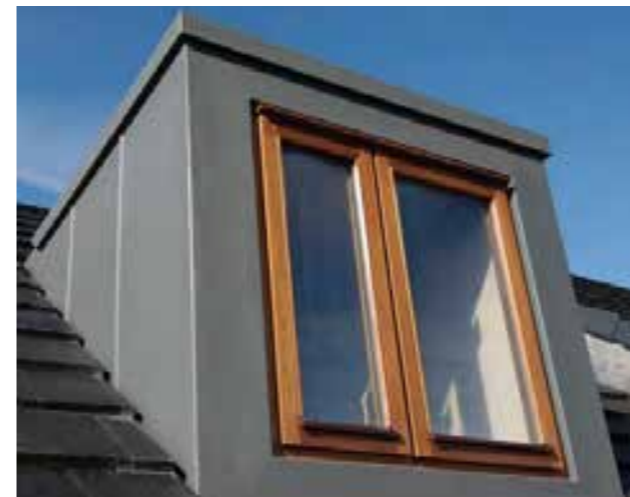
Lead clad dormers
