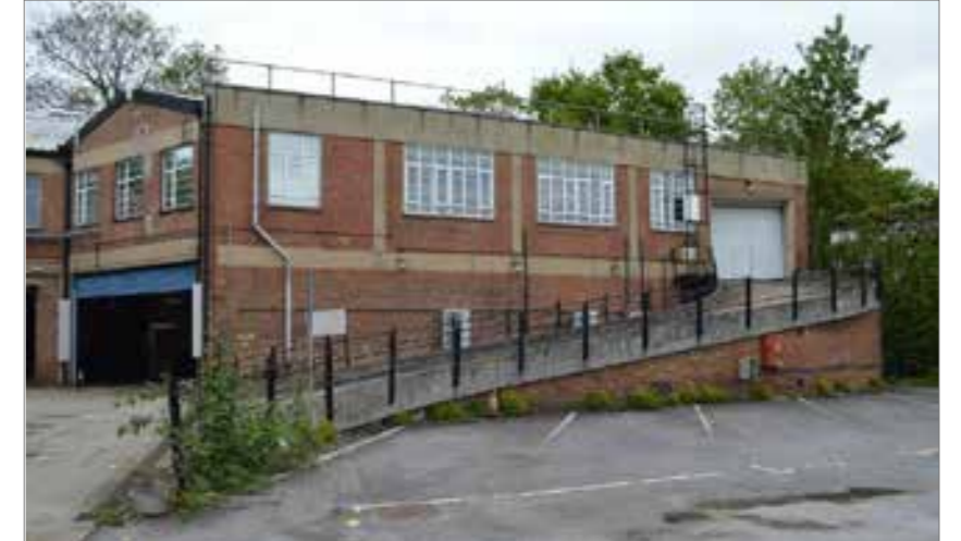
The garage and ramp at the rear of the site
