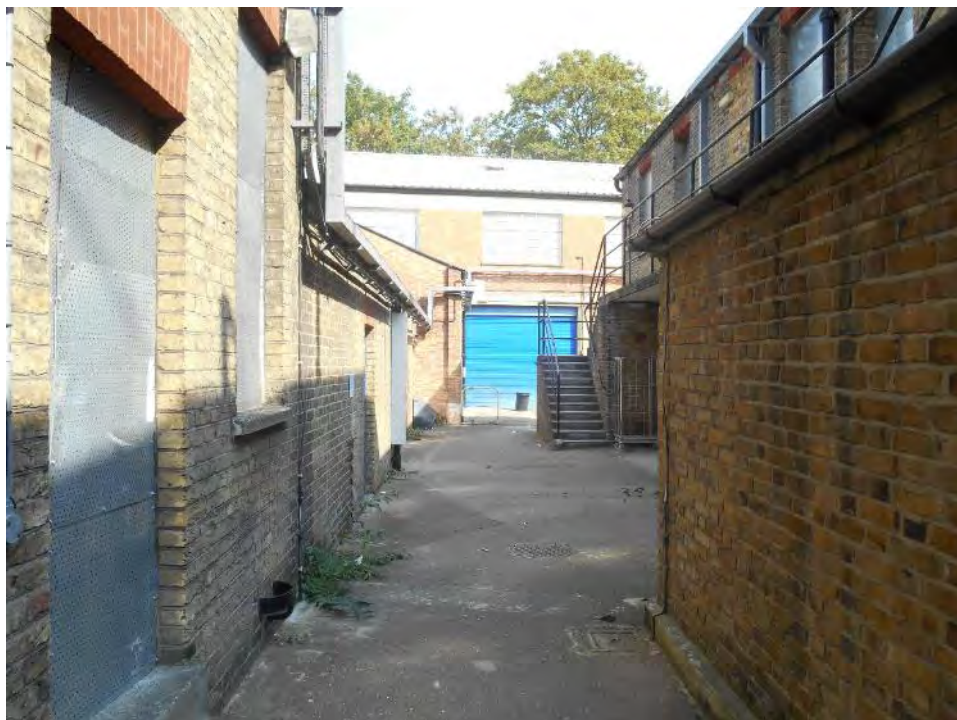
Photo 26: Back of the Police Station building
