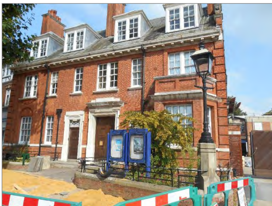
Photo 10: View of Police Station from Station road
