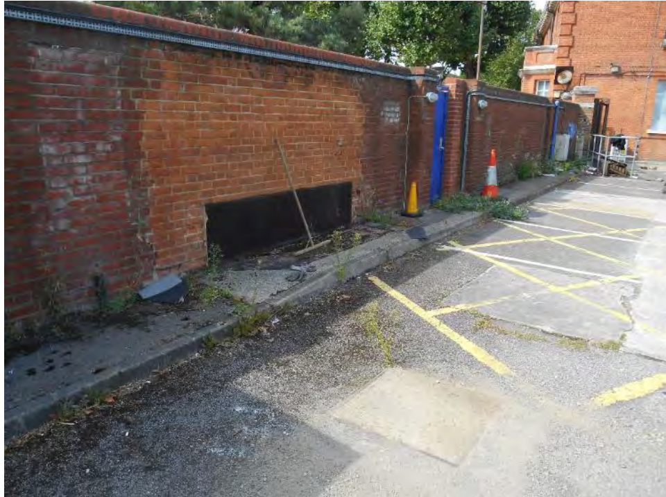
Photo 29: Location of the two large underground tanks and one smaller tank
