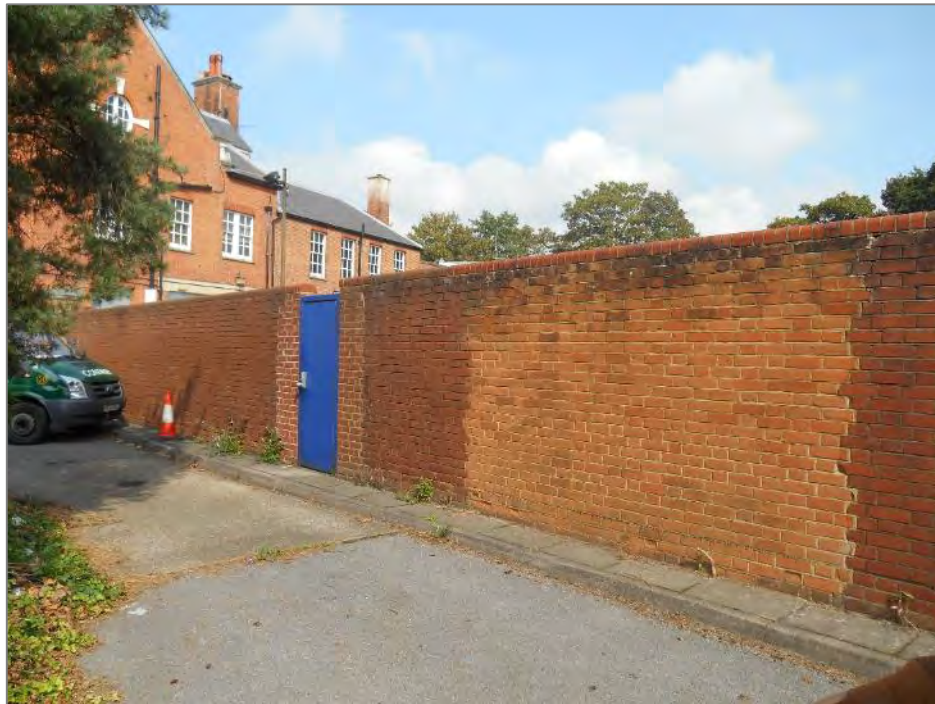
Photo 11: Front of Police Station
