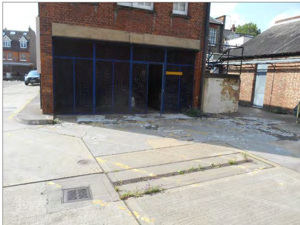
Photo 22: Location of the two smaller underground fuel storage tanks located at the rear of the station
