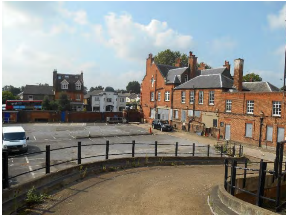
Photo 27: View from ramp
