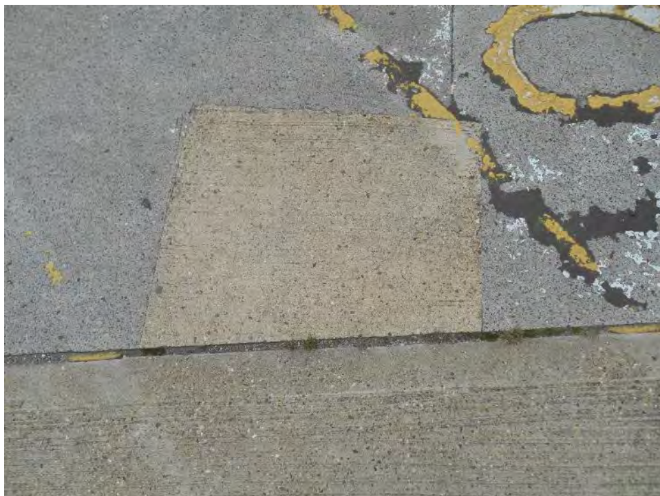
Photo 36: Underground fuel storage tank located at the rear of the station
