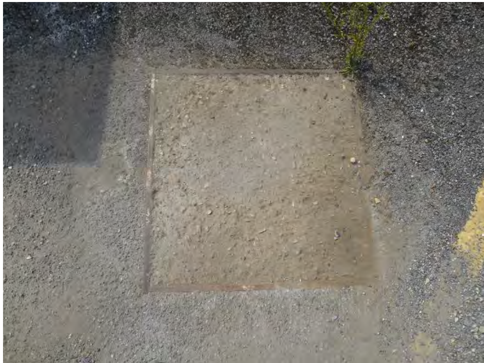
Photo 30: Underground tank located at the front of the station
