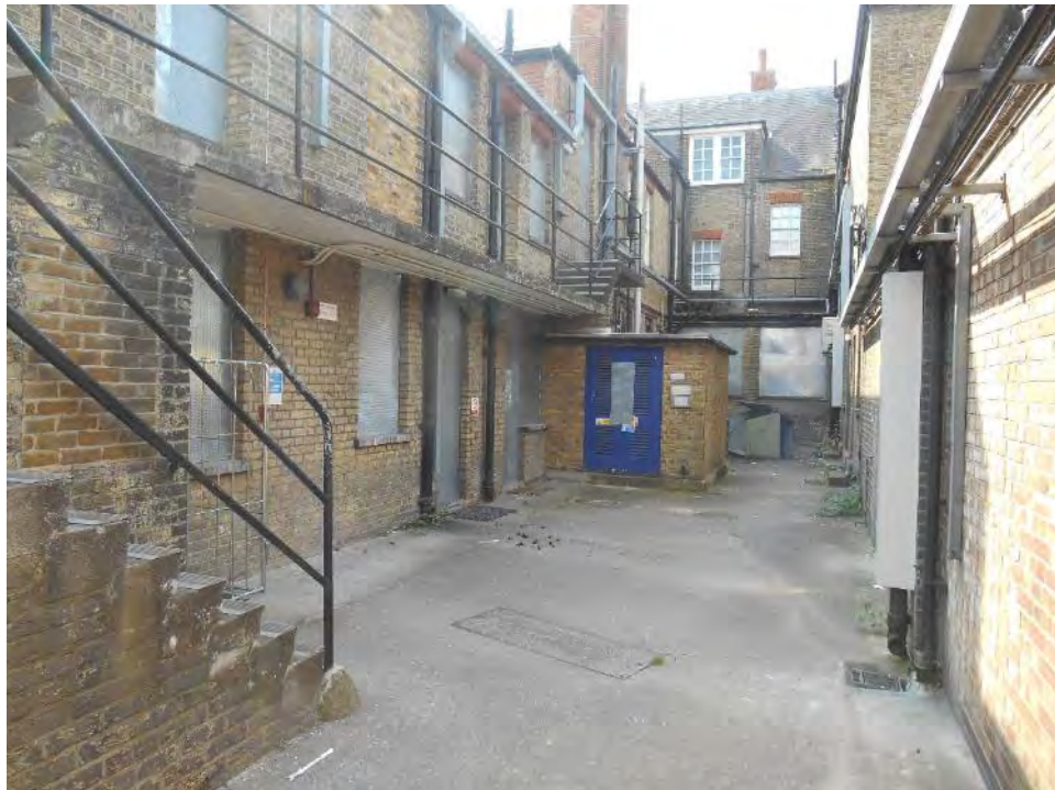
Photo 24: back of the Police Station building
