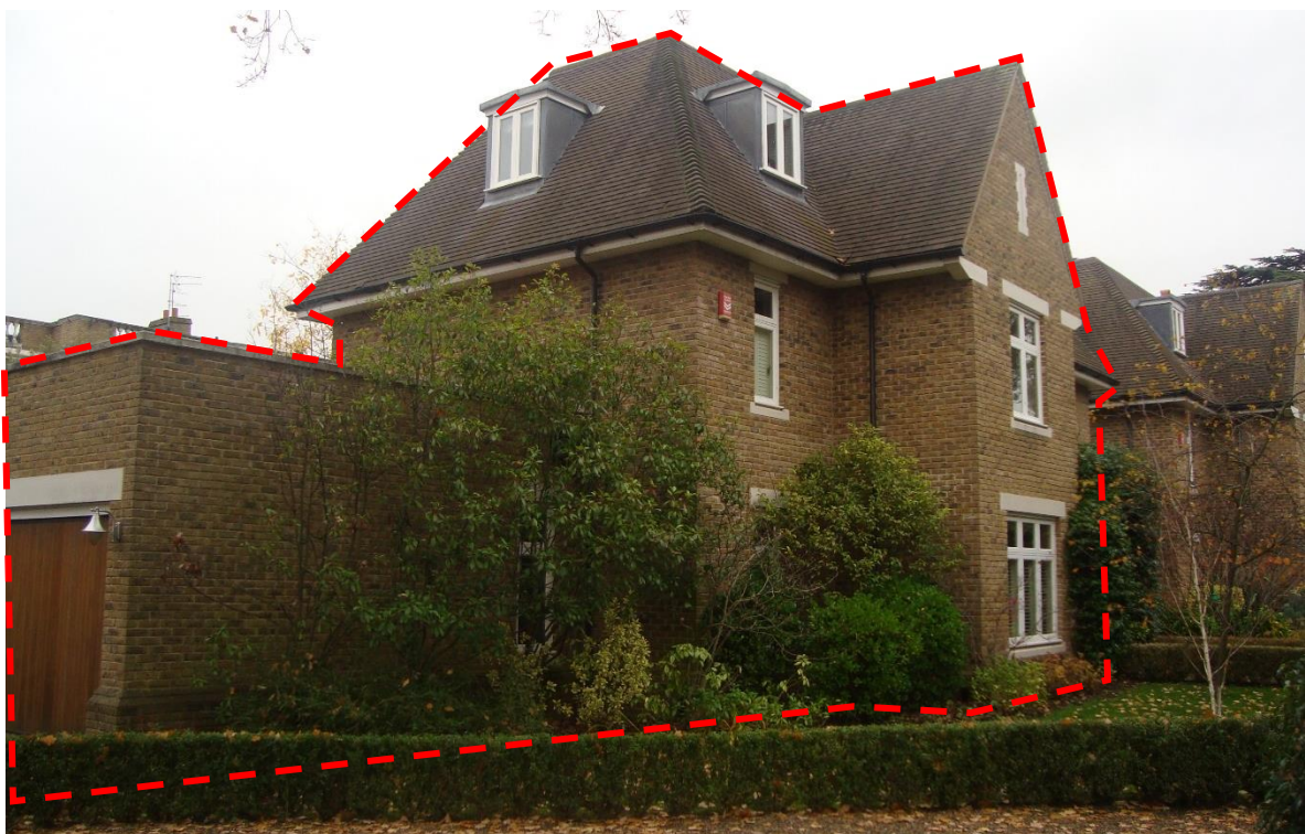
Figure 2 – View of the front of the property as seen from the junction between Chalmers Way, Corsellis Square and Varley Drive
