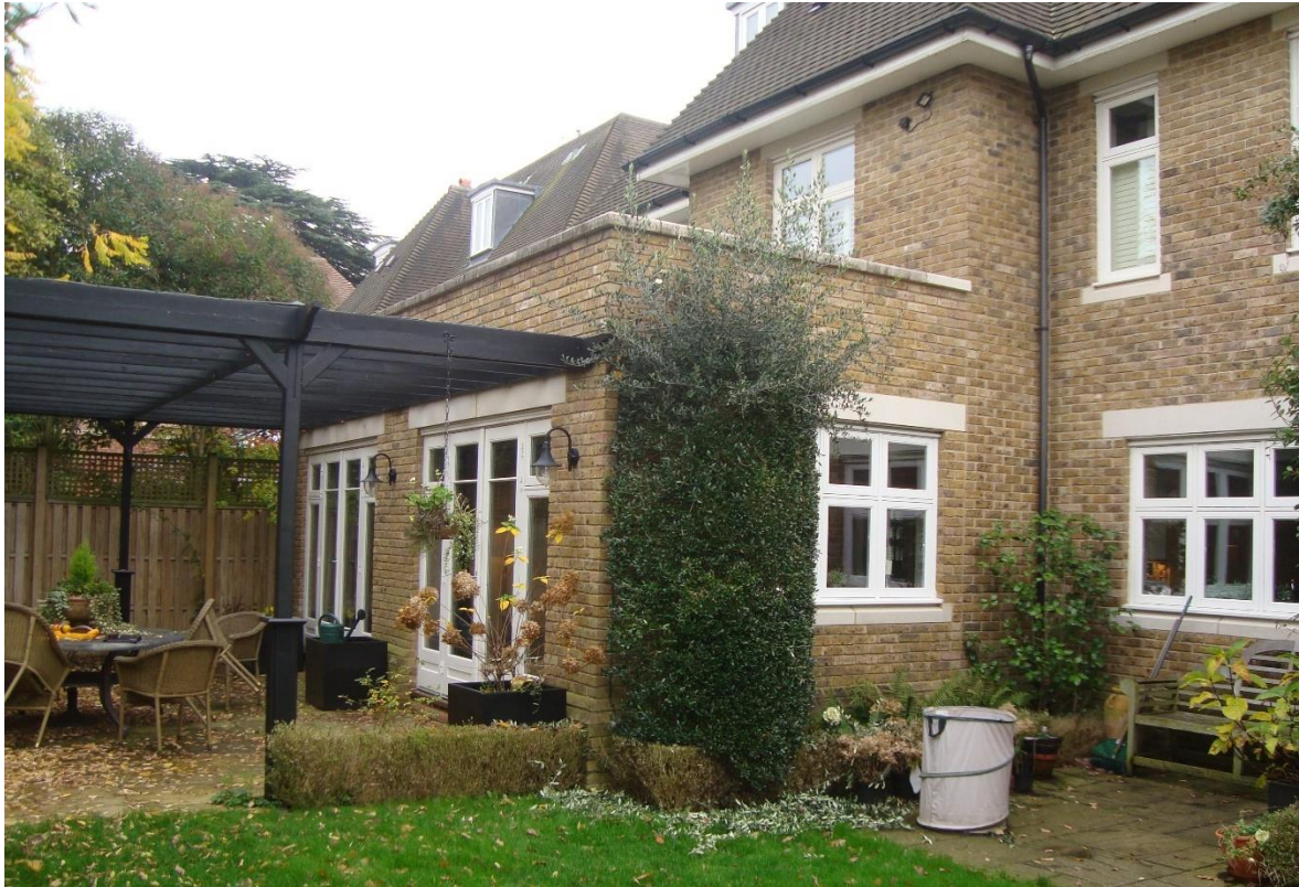
Figure 11 – View of the existing rear elevation as seen from the garden.
