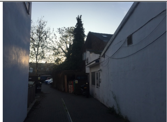
Photo 4: Building B1 with Building B1 and B2 attached at second storey level.
