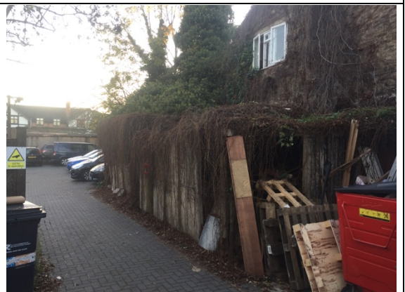
Photo 6: Building 2 showing the virginia creeper and building 5.
