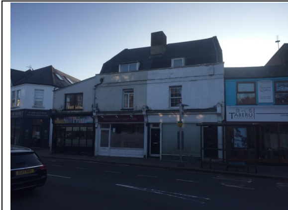
Photo 1: North-eastern elevation of Building B1 that is adjacent to the High Street.
