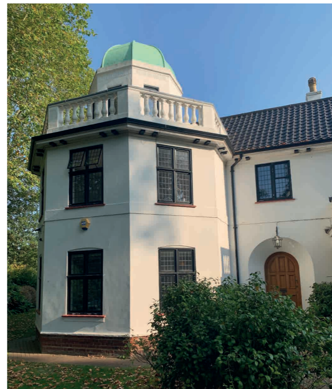
Photograph of Existing Roof Tiles
