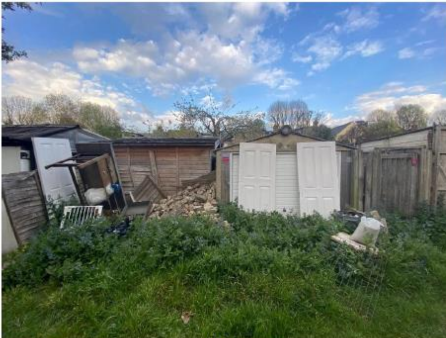
View from the rear lane looking back at the garage
