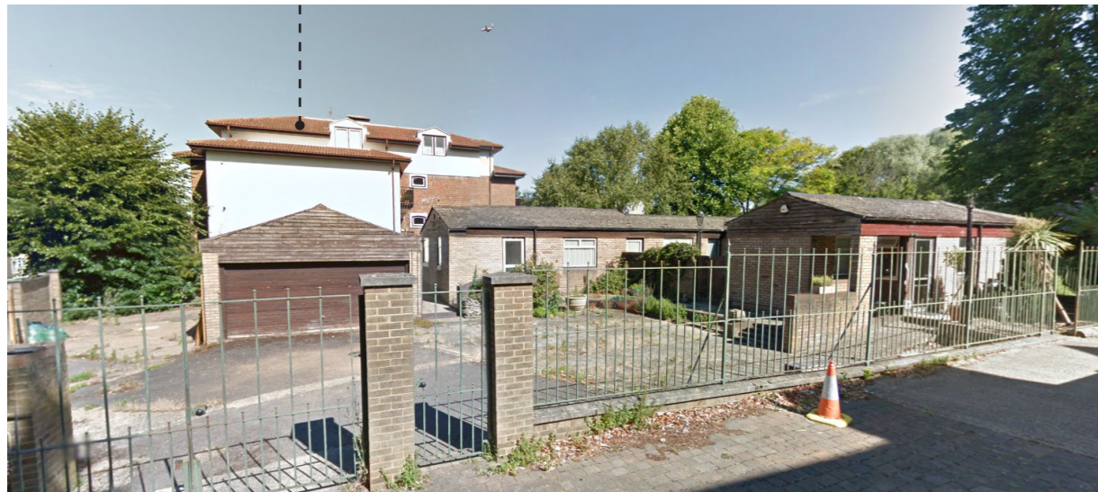
Street view of The Bungalow and Annex
