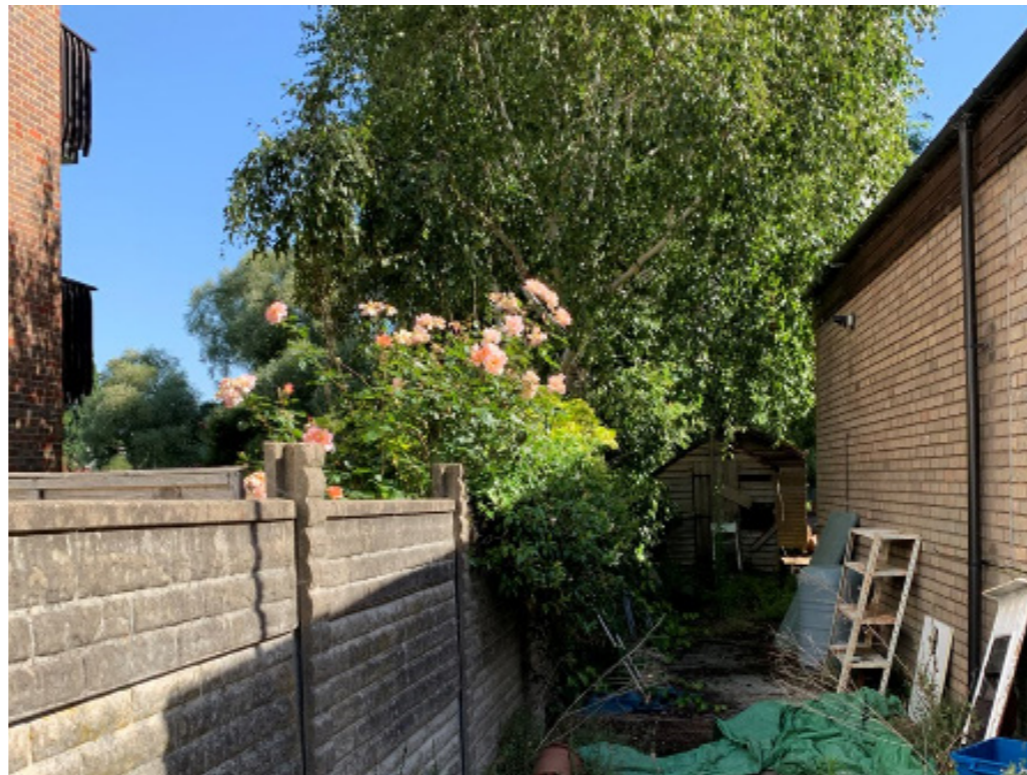
Western Boundary wall
