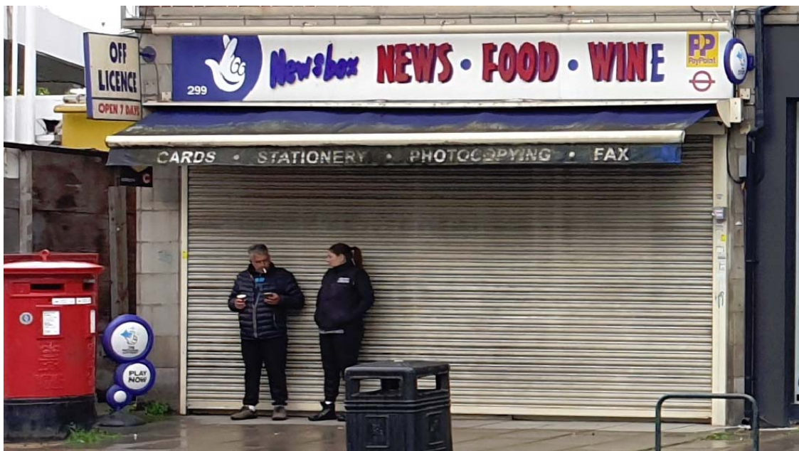
Fig 1. 299 Richmond Road fully enclosed external shutter to shopfront.
