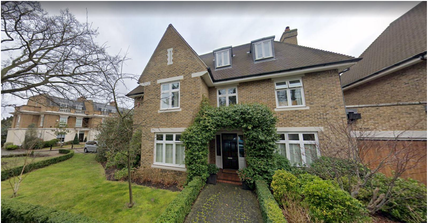
Figure 5 – View of 20 Chalmers Way front elevation
