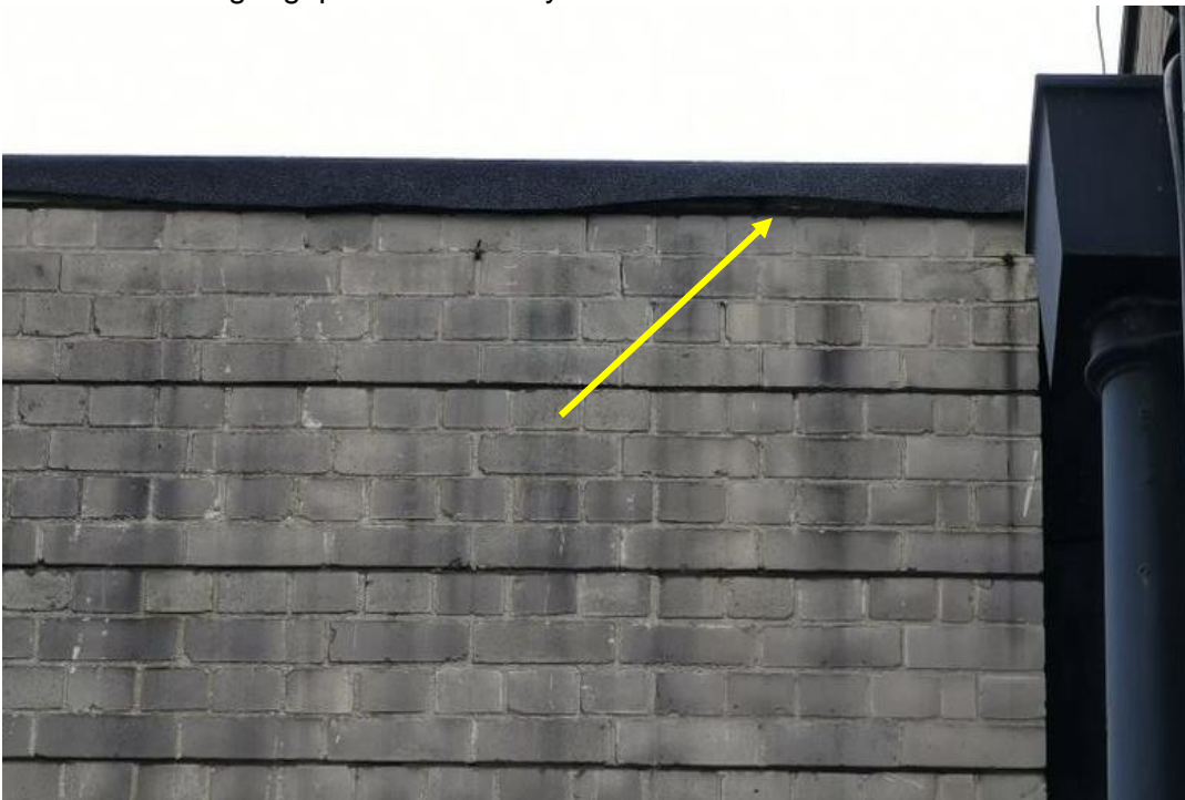
Plate 4: showing a gap under the felt yellow arrow.
