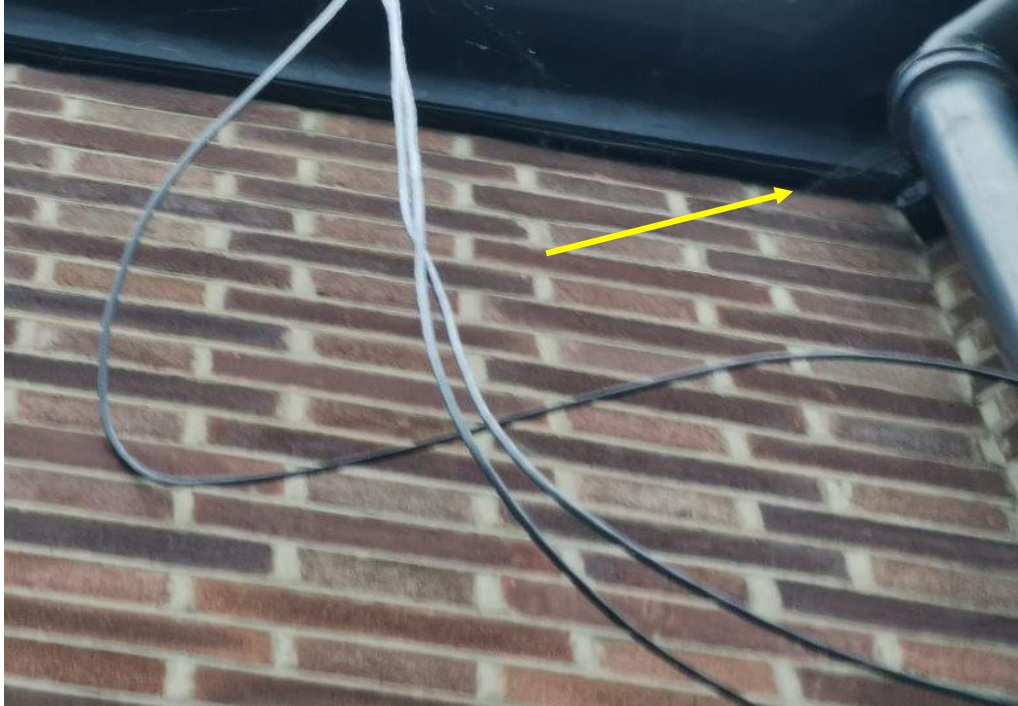
Plate 2: showing gaps under the wooden panelling
