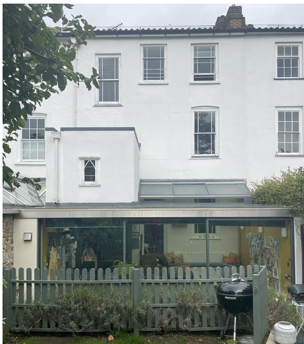
Figure 3. Current rear elevation illustrating altered sash windows
