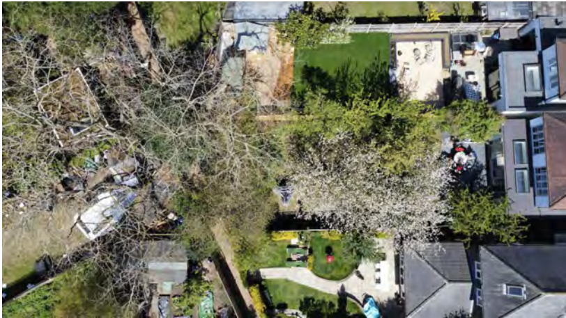
Photographic plate showing an aerial image of the survey site.
