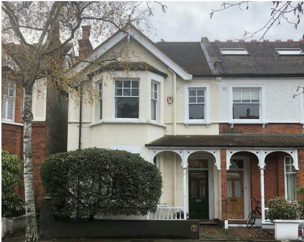
FRONT ELEVATION FROM ACROSS THE STREET
