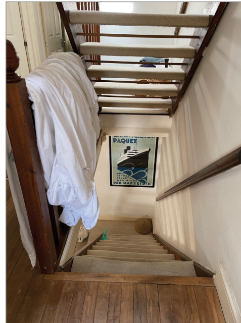
Stairs to First Floor 03
