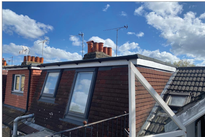
Neighbours roofs (26, 28 Rosedale Road)
