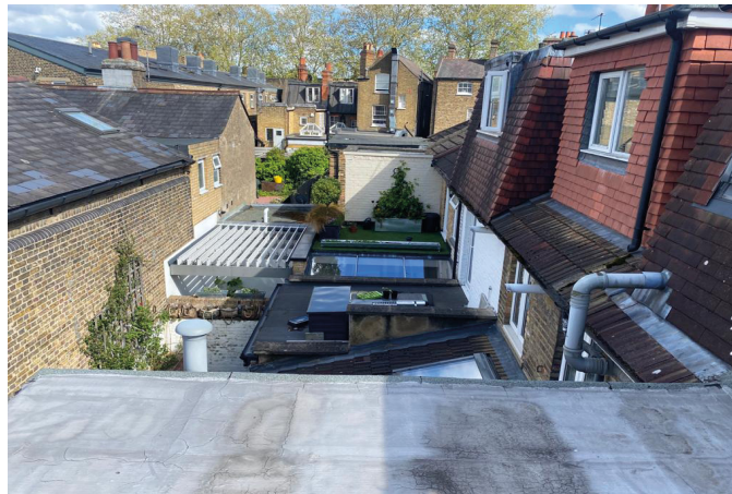
View East from Rear Terrace 13
