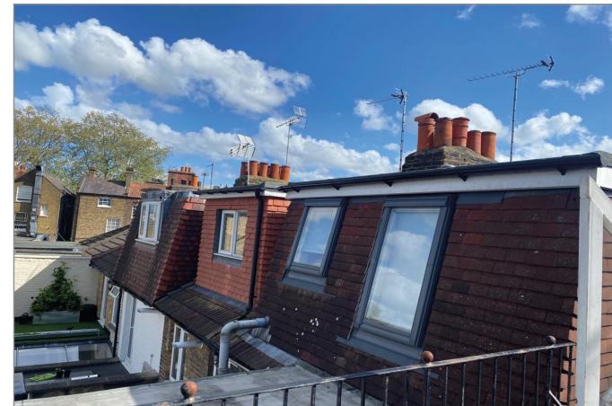
Neighbours roofs (26, 28, 30 Rosedale Road)
