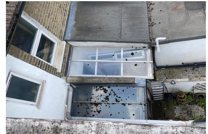
Viewing lower roofs 14
