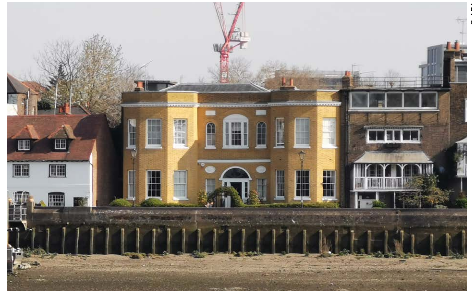
Fig. 22: No. 10 Lower Mall (Kent House)
