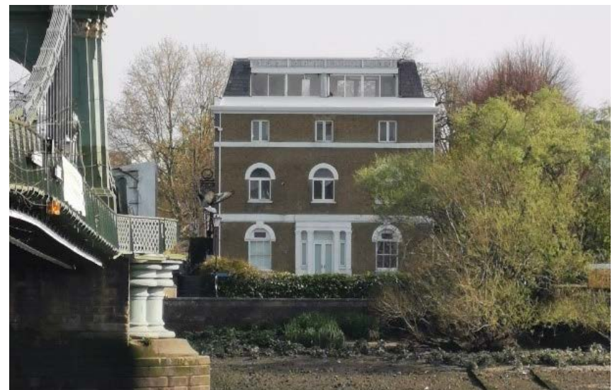
Fig. 32: Nos. 107-109 Hammersmith Bridge Road, view from the southern Thames Path
