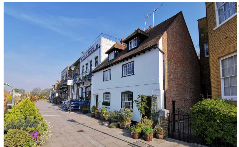
Fig. 23: Nos. 11-12 Lower Mall
