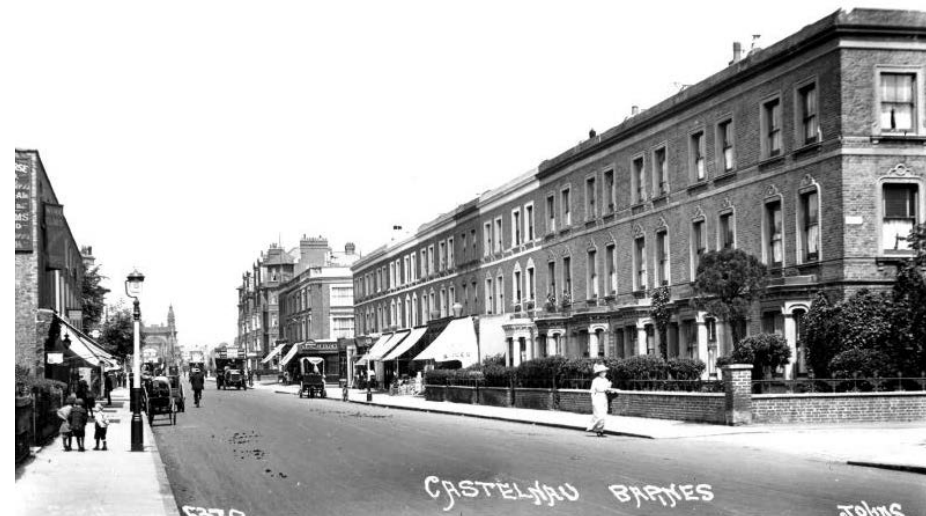
Fig. 37: View north along Castelnau, c.1900
