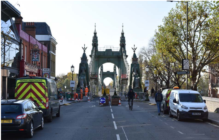
Fig. 52: View south down Hammersmith Bridge Road, 2020
