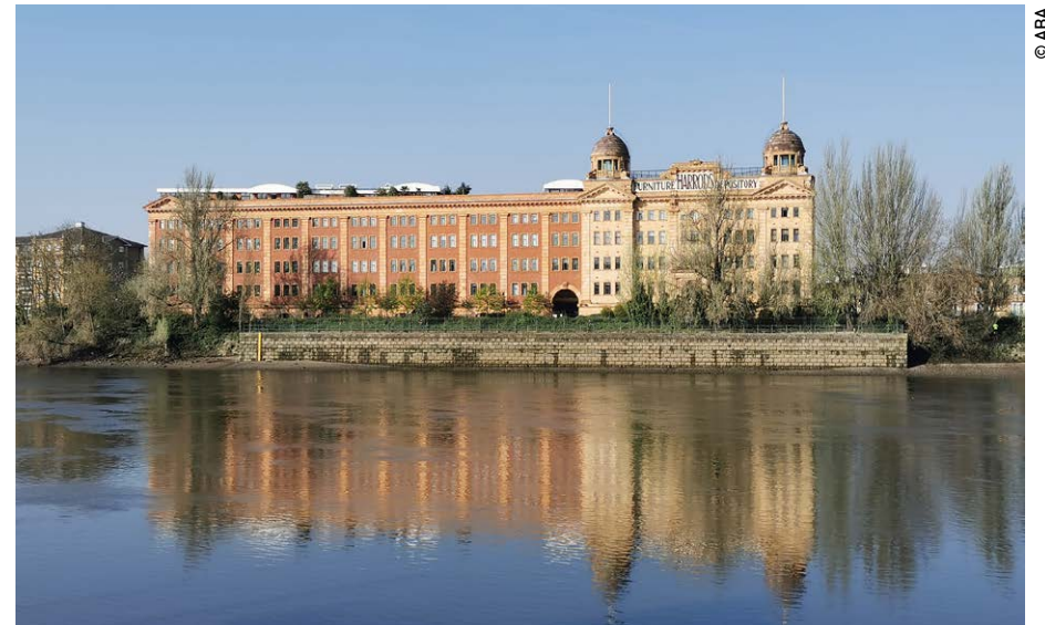
Fig. 41: Grade II listed former Harrods warehouse viewed from the north bank of the Thames
