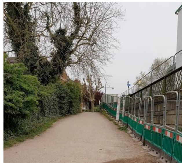
Path to the Side of Hammersmith Bridge
