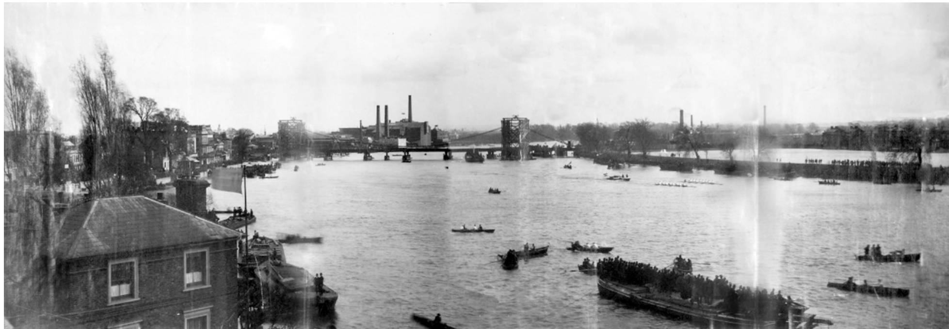
Hammersmith Bridge under construction 1886
