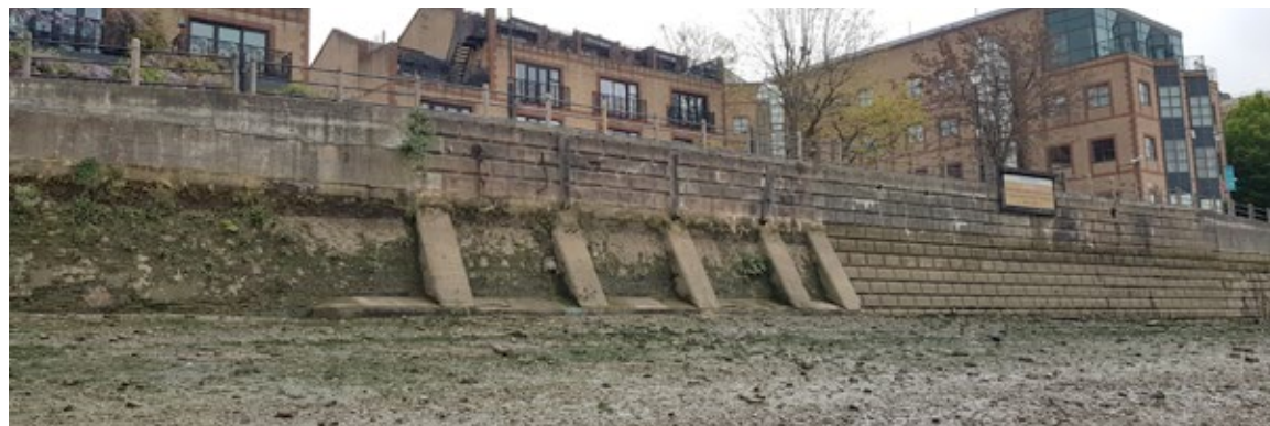
Buttressed Flood wall at Chancellor's Wharf
