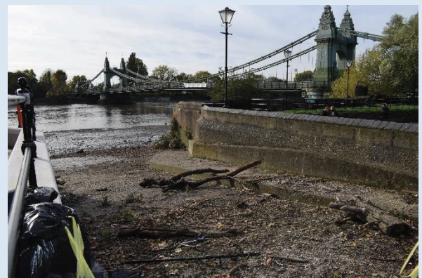
Looking southwest from the Queen Caroline Street flood gates. The corner river wall in centre frame will accommodate the northern abutment of the proposed temporary bridge with the bridge ramp extending rightwards along the river wall before meeting the ground at street level.
