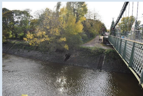
View from Hammersmith Bridge looking southwest to Barnes and the landing area and southern abutment of the proposed temporary bridge in centre frame.
