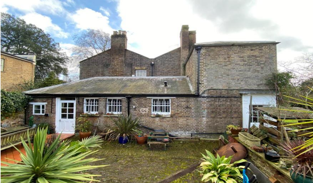
Fig. 24: View, looking south, of the north elevation, with No. 1A in the foreground and the later phase of Riverside House proper, immediately beyond.
