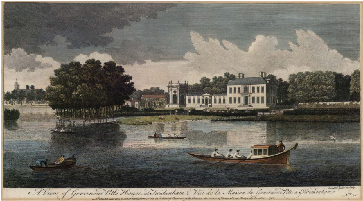
Fig. 5: John Boydell, A View of Governour Pitt's House in Twickenham , 1753 (Orleans House Gallery)
