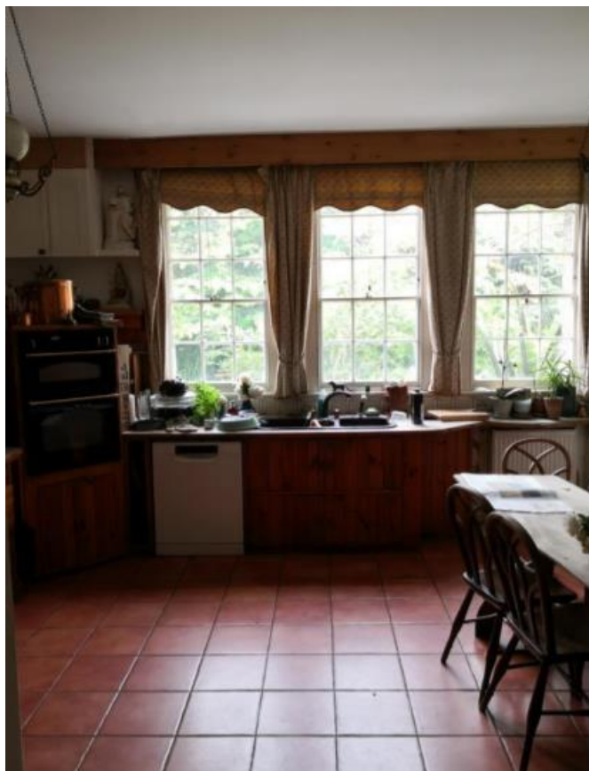
Fig. 20: The existing kitchen of Riverside House, to be converted to living-room space for No. 1A.
