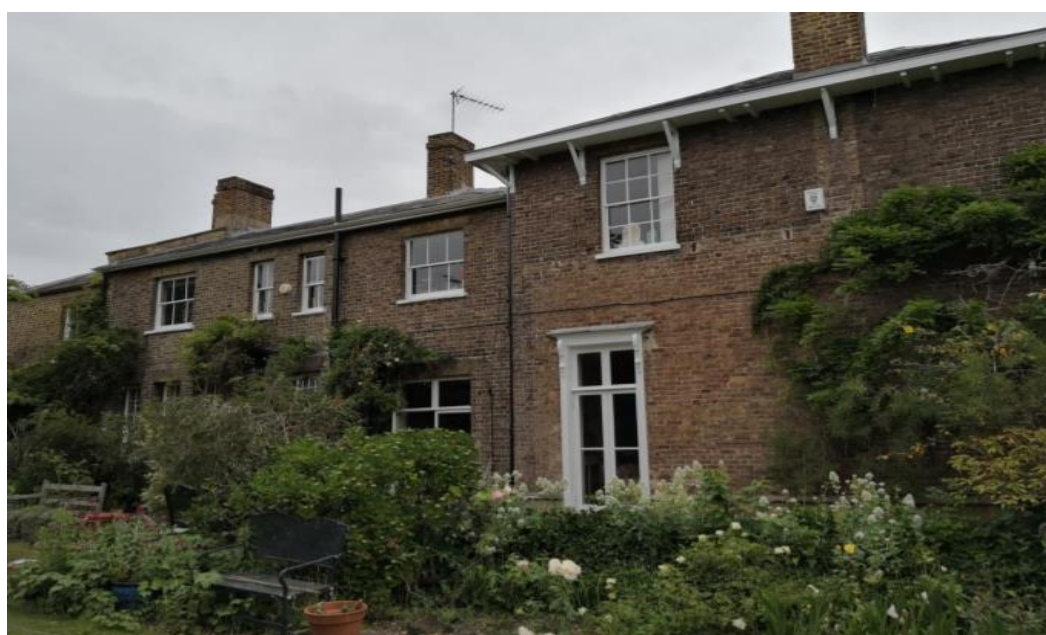
Fig. 23: View, looking north-east, from the garden of Riverside House, showing clear external distinction between the earlier 'cottage' building (left) and the c. 1810 extension (right).
