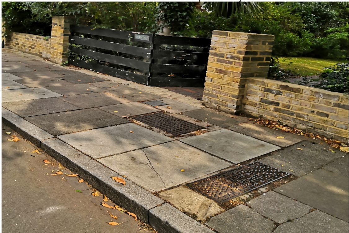
Manholes on the pathway
