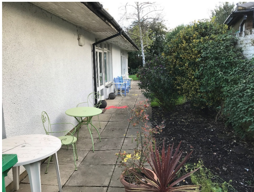
Description: Elleray Hall Site.
