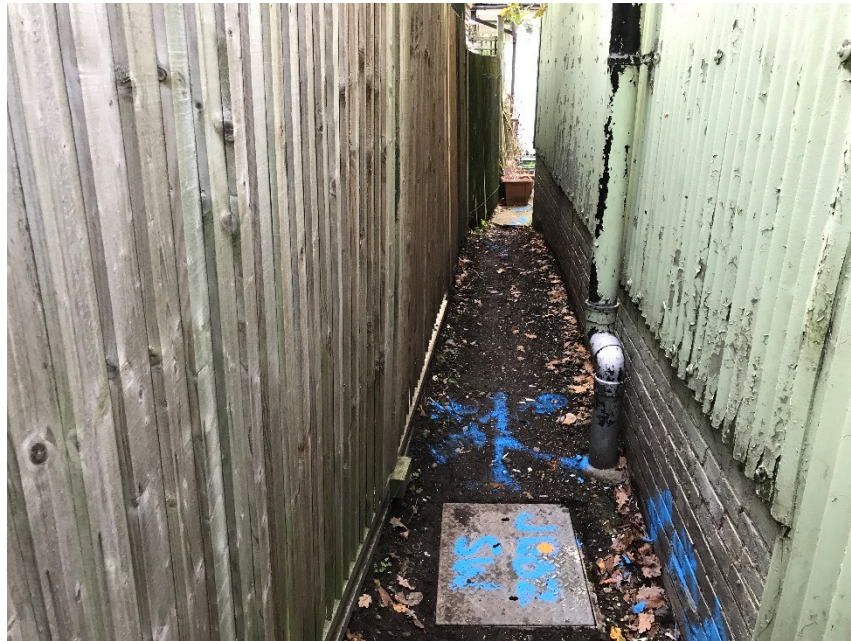
Description: Elleray Hall Site.
