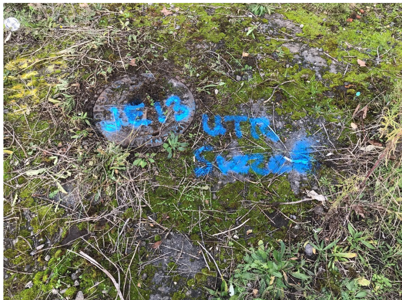
Description: Manhole JE13 UTR Seized.
