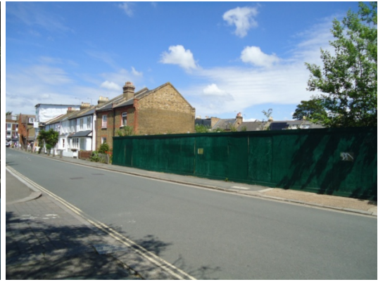
Site 1 frontage to North Lane
