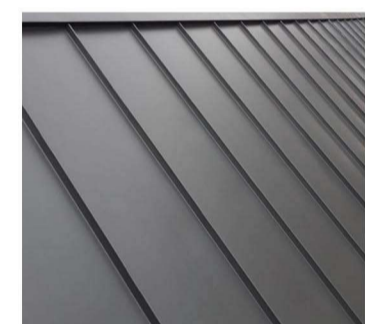
Light grey standing seam metal roofing
