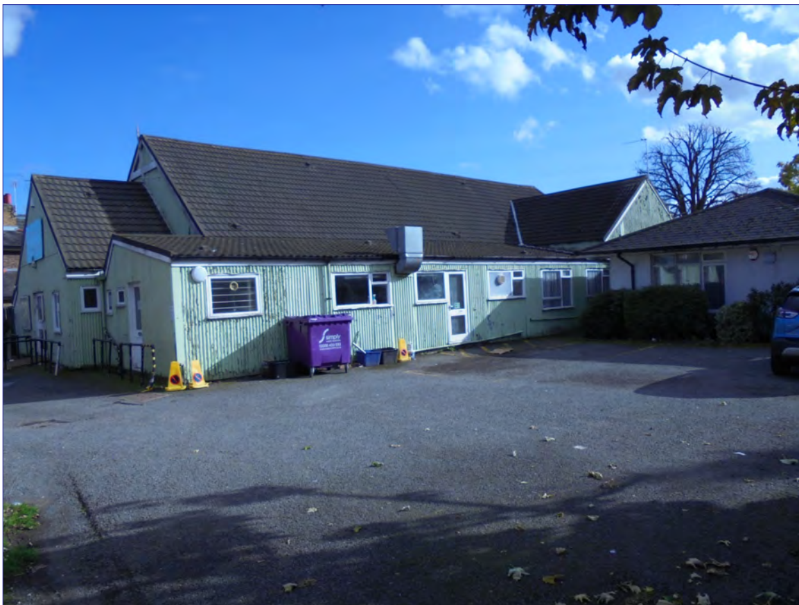
Plate 10: Southeast facing view towards Elleray Hall
