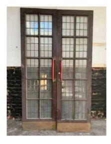
New entrance door to match with the surrounding area and the existing features. The door it is already on site and will be restored in order to re-use original elements of the building. The glazing units will provide the light needed into the communal entrance hall of the proposed development.
