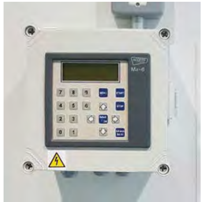
▲ An example of a wall mounted control box used in conjunction with an automated irrigation system
