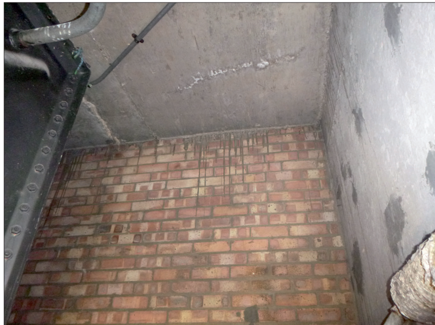
Photograph 3: Showing the well-sealed service unit.
