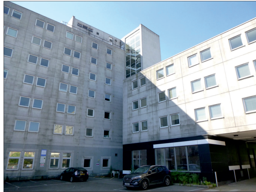
Photograph 2: Showing the rear of the building.
