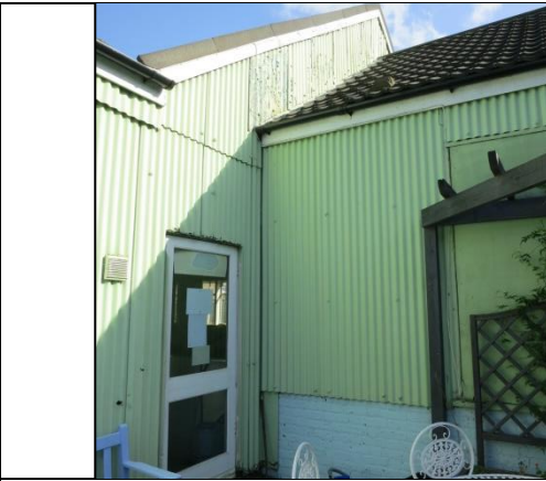
Photograph 10: Hardstanding to the west of site 1
