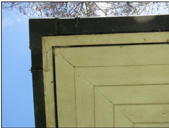
Photograph 17: Gap in soffit of B1b.
