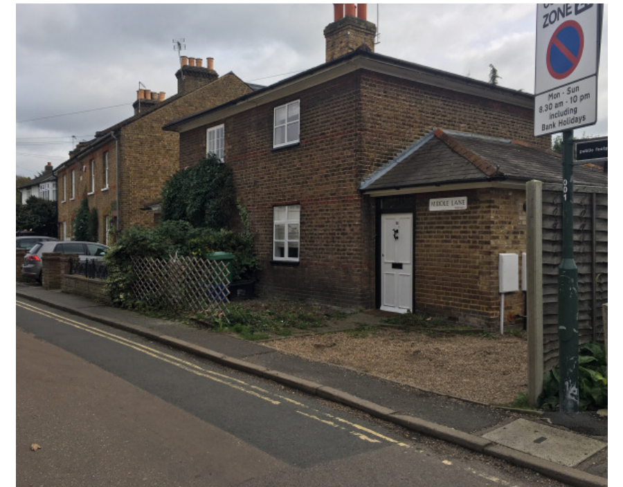
VIEW OF 15 MIDDLE LANE, EAST OF ELLERAY HALL
