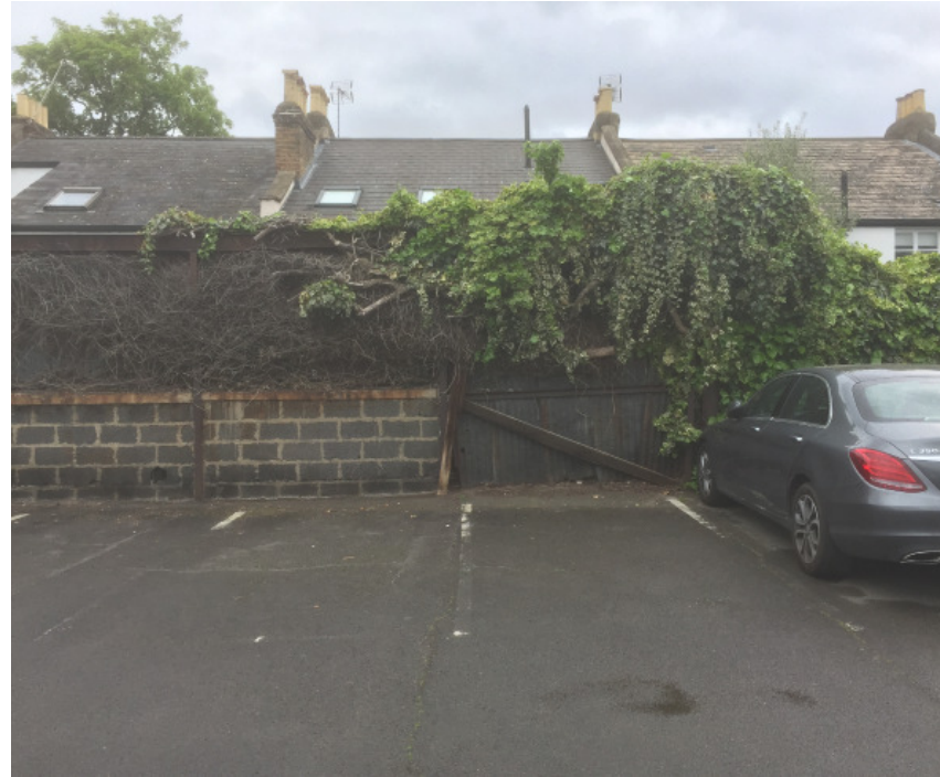
EAST CAR PARK SITE LOOKING EAST
