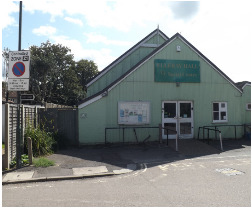
ELLERAY HALL EXISTING FRONT ELEVATION
