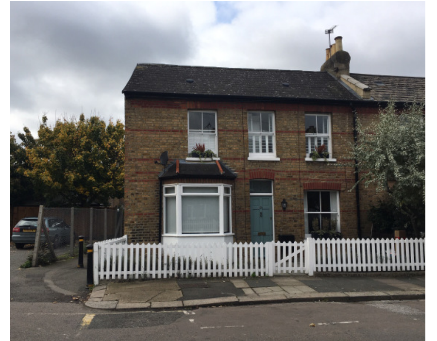
VIEW OF 26 ELLERAY ROAD LOOKING WEST
