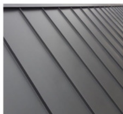
Light grey standing seam metal roofing
