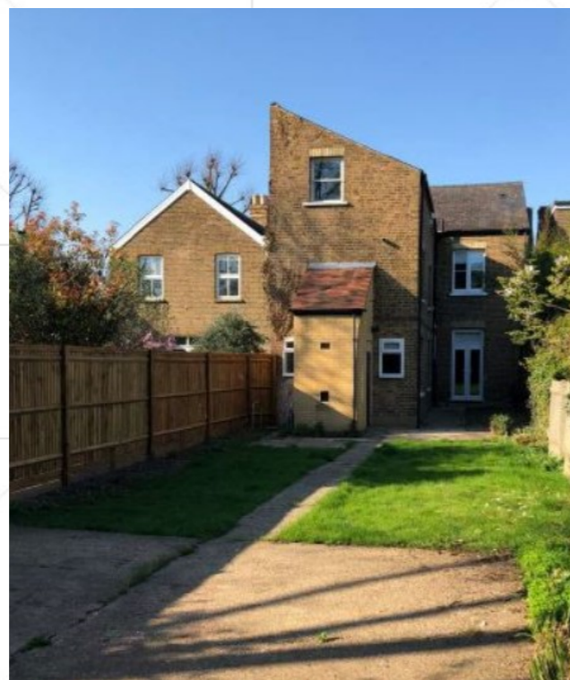
Figure 4: Existing rear elevation
