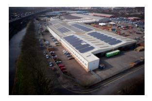
Panel Model999 x ET Solar 250WInverter Model8 x PowerOne TRIO-27.6-TL,<br/>1 x PowerOne PVI-10.0-TLMonitoring<br/>SystemPower One AEC EVOSystem Size250 kWpAnnual Output202,174 kWh/year
