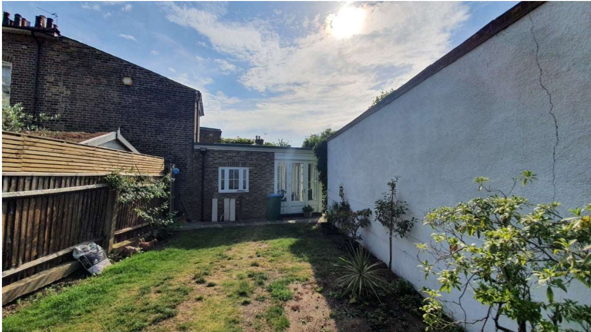
Image 009: View looking West from site of proposed garden room back to 165 Richmond Road. Marble Hill Close garages to right of image, 167 Richmond Road to left of image.
