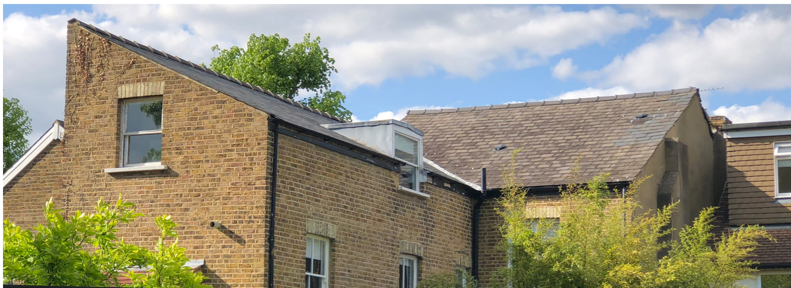
FIGURE 05 - EXISTING REAR ROOF AND OUTRIGGER
