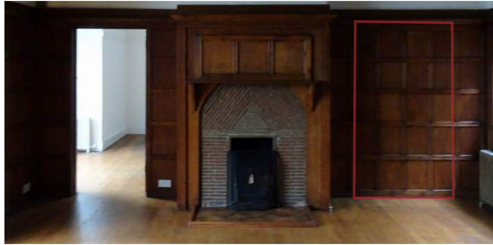
14. Existing panelling to Music Room (rectangle indicates new opening)
