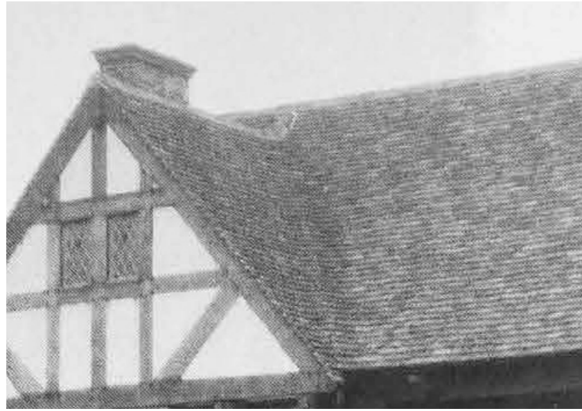
28. Original swept verge and ridge tiles of the roof
