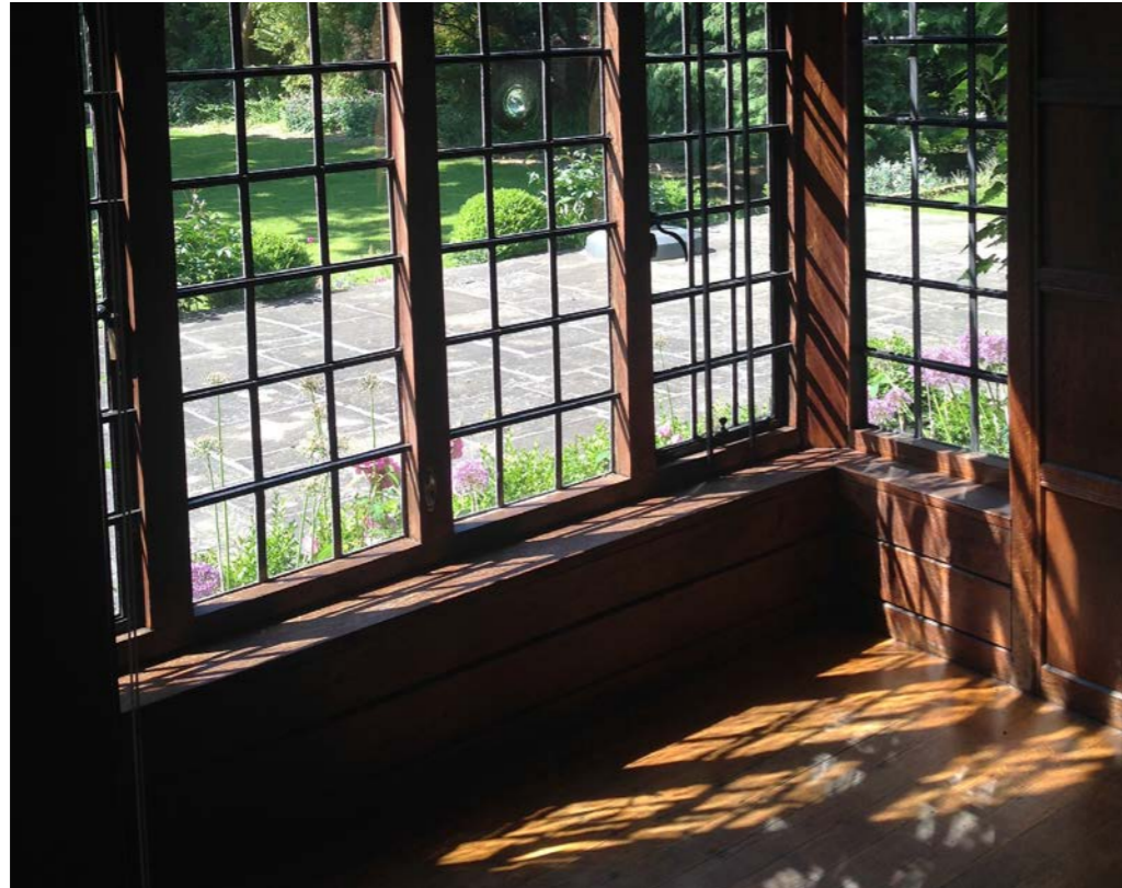
29. Existing bay window of the Music Room
