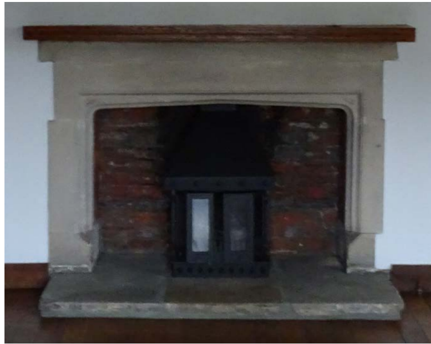
11. Existing fireplace in the Study, showing modern raised concrete hearth
