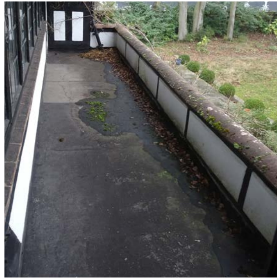
20. Existing first floor terrace
