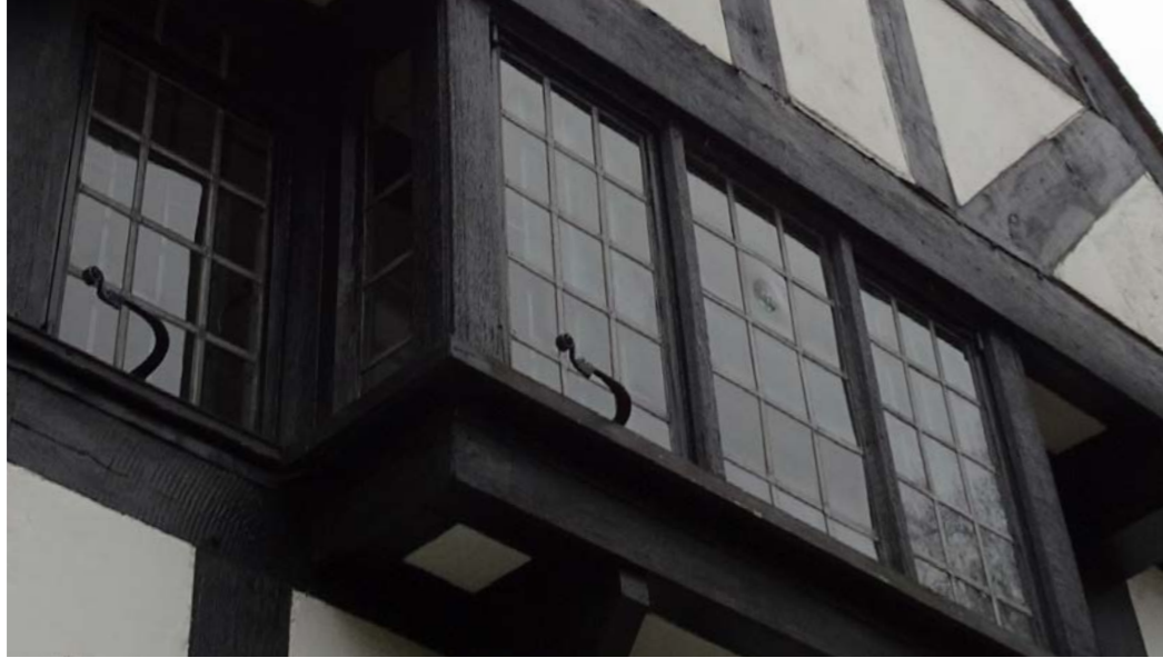
6. Original metal casement timber-framed leaded lights
