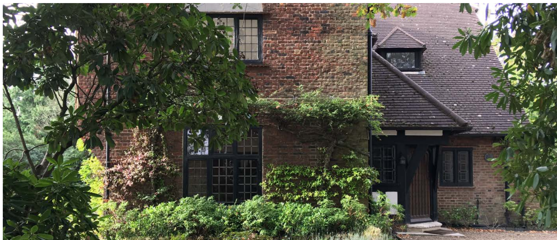
3. Sheengate view from east
