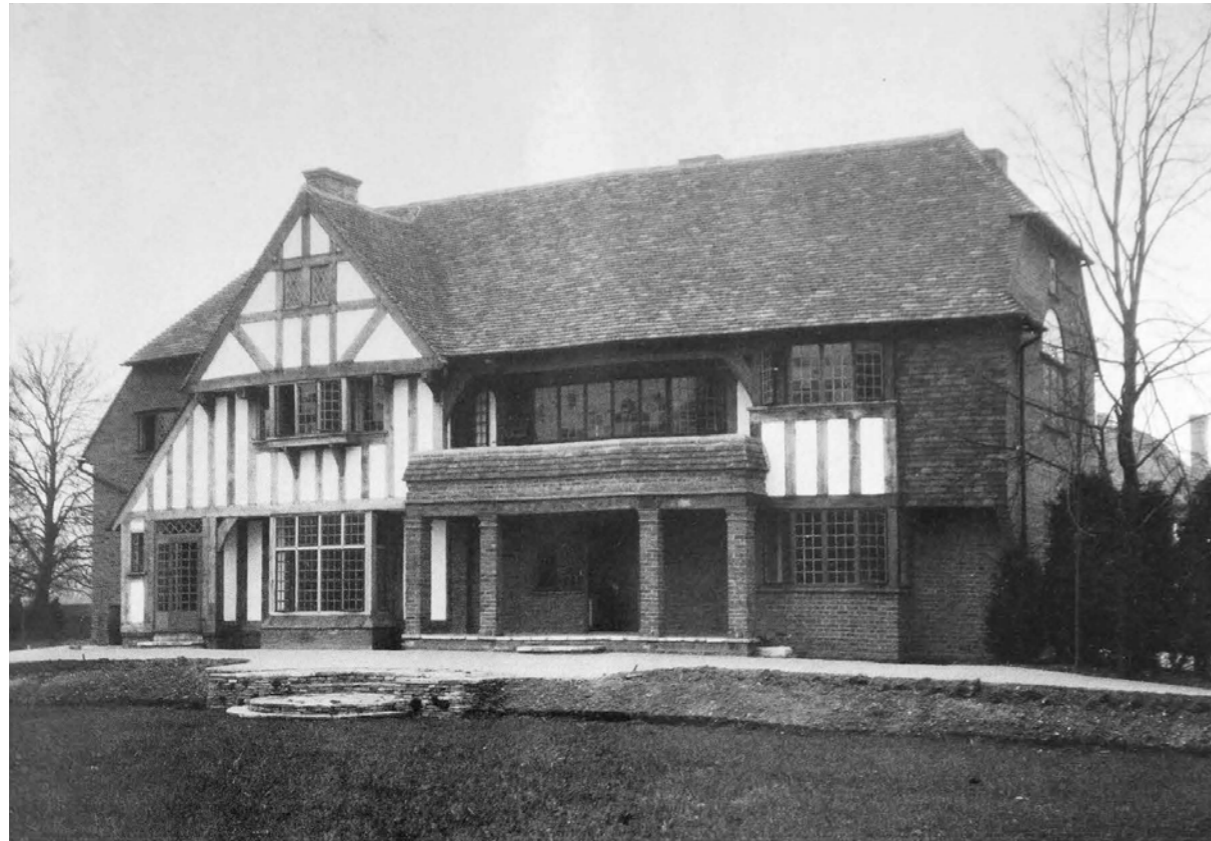
7. Original photograph of Sheengate c.1925 showing natural finish to all external timber
