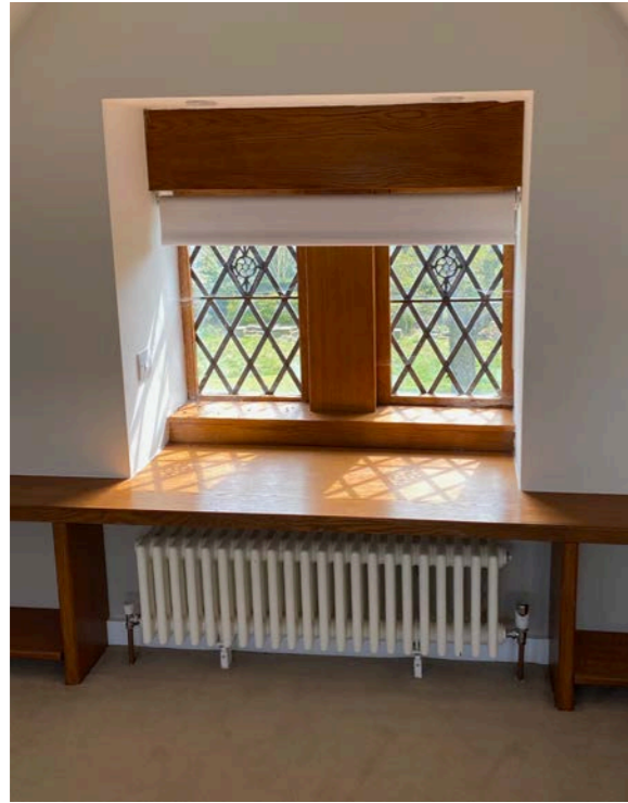
22. Modern timber lining to be removed
