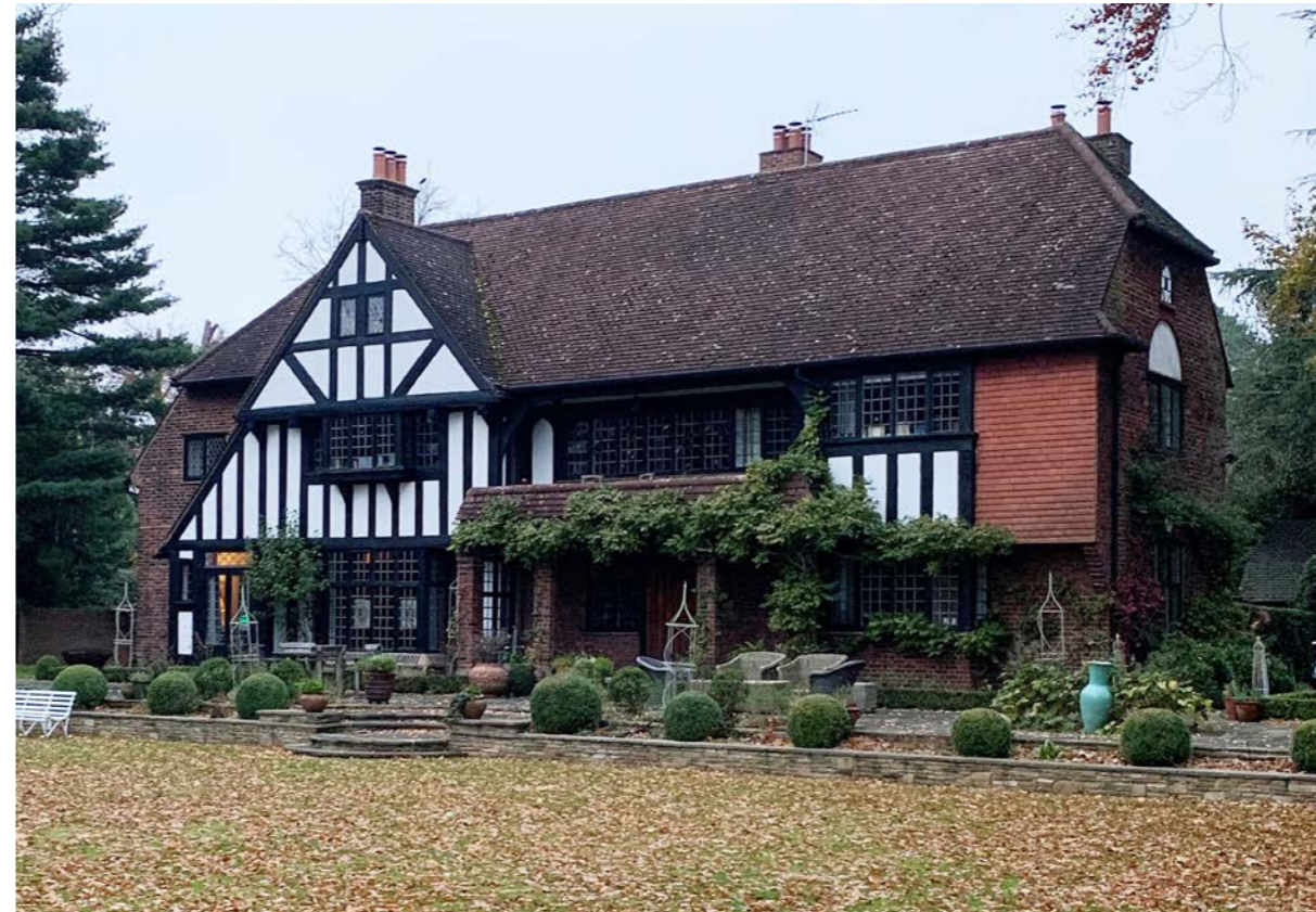
8. Photograph of Sheengate in 2021 showing black stained timber frame and windows
