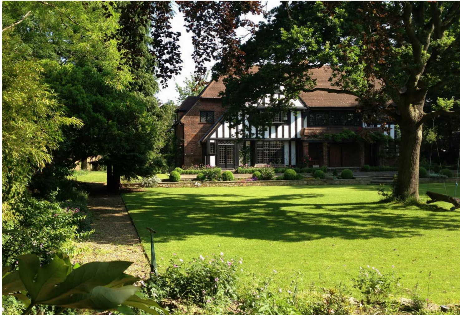
2. Sheengate view from south
