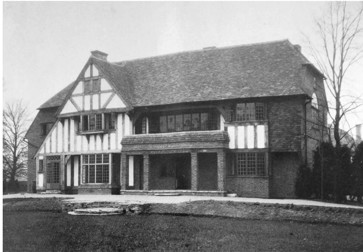
5. Original photograph of Sheengate c.1925 showing natural finish to all external timber
