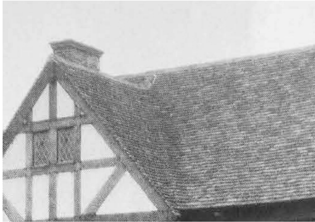
9. Original swept verge and ridge tiles of the roof
